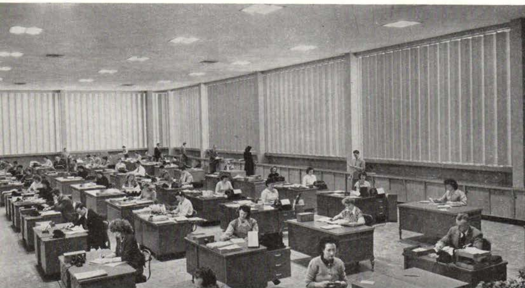
Among several types of inside sun control devices are vertical metal louvers. Those illustrated here are in the general office area of the Guarantee Insurance Company, Los Angeles. Photo: Woro Studios
