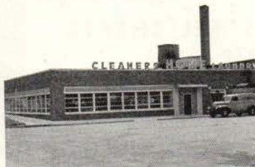
Laundry—Laundry, Bloomington, Indiana. Contractor: Harlos Building Service.
