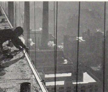
Stainless steel spandrel flashing at all floors
