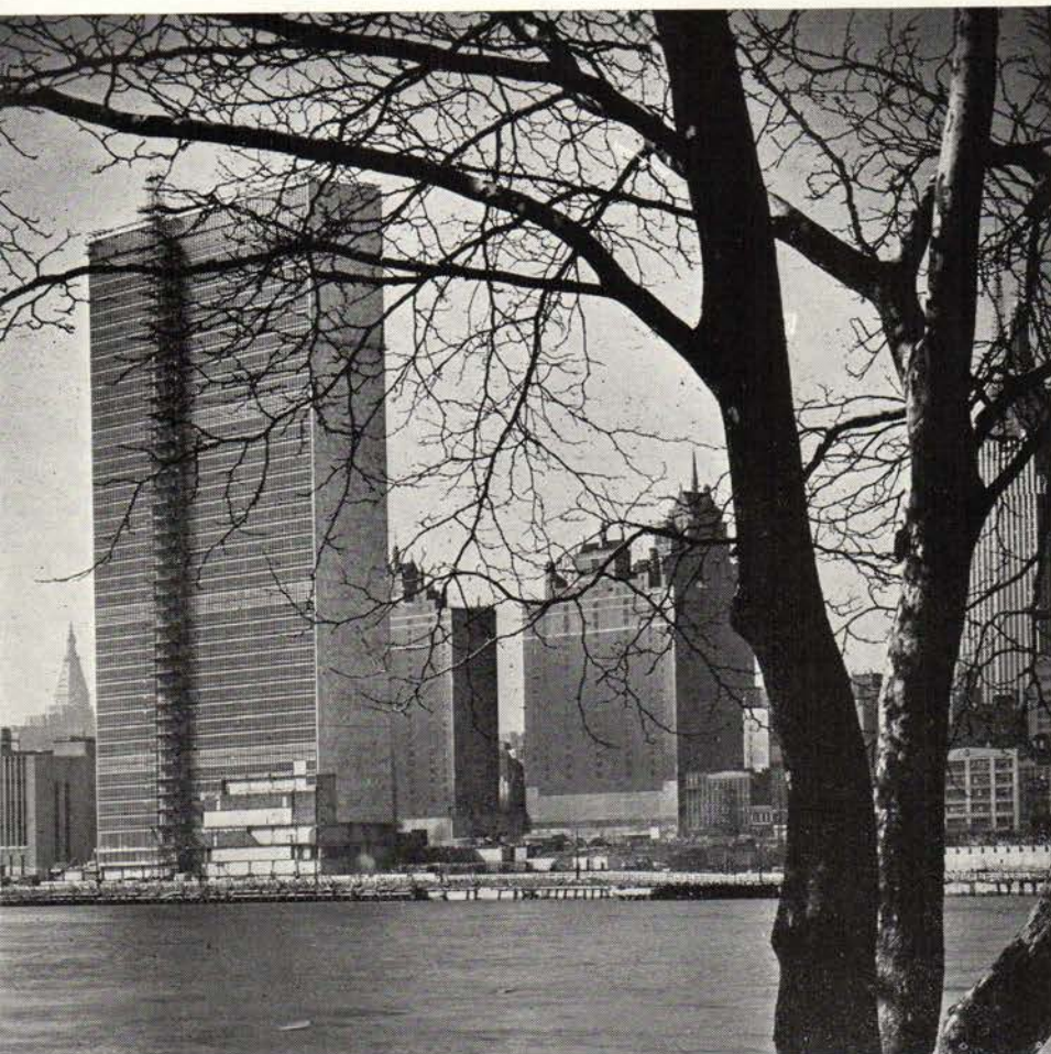
Left: the eastern side of the building, viewed from Welfare Island in the middle of the East River. The vertical line is a construction hoist.
