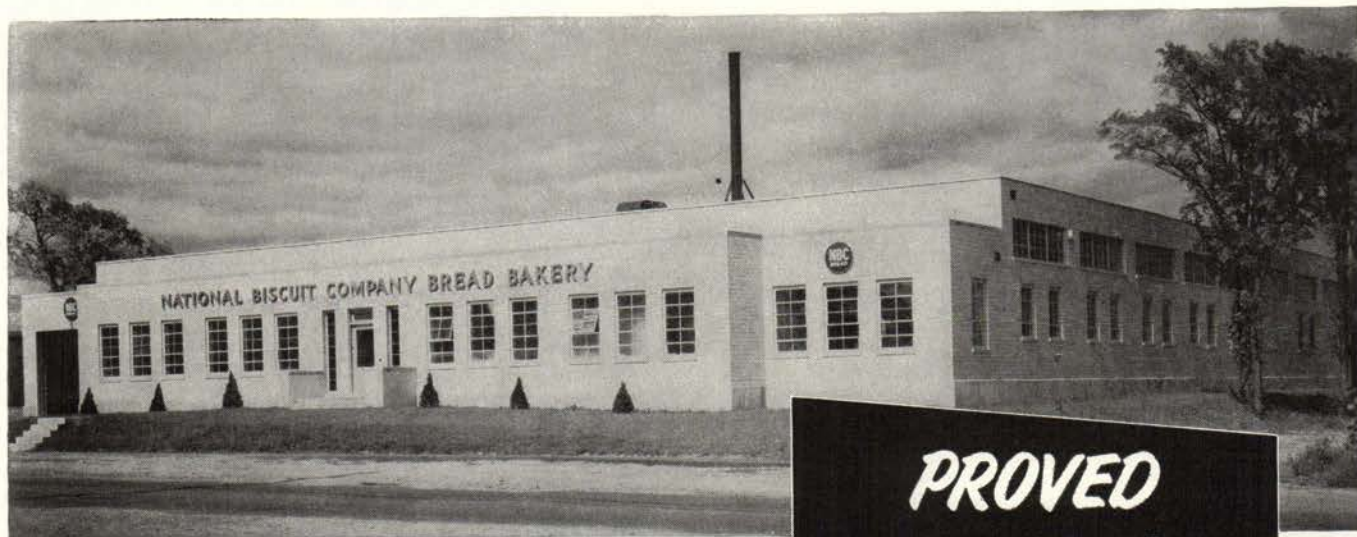
National Biscuit Company Building, at Plattsburg, New York. Natco Manganese Spot Dri-Speedwall Tile for Exterior Walls. T-series Ceramic Glaze Vitritile for Interior Walls. Contractors—Wright and Morrissey.
