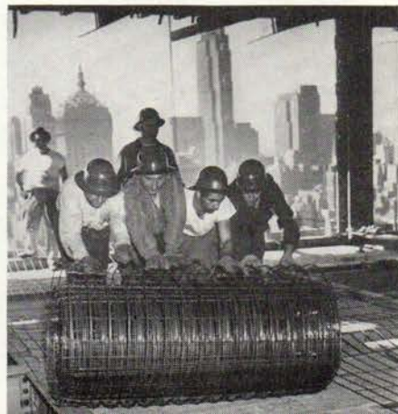
Welded wire mesh for floor-slab reinforcement
