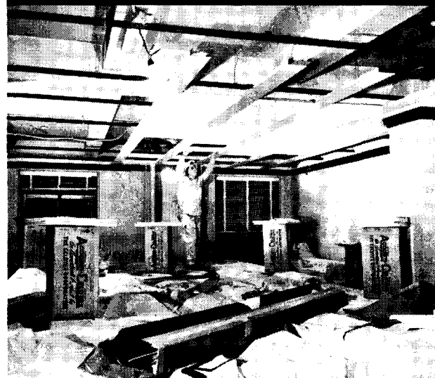
Metal Panels are Quickly and Easily Secured to "Grid" with Metal Clips—Perfect Alignment Assured. Acoustical Material Rapidly Positioned
