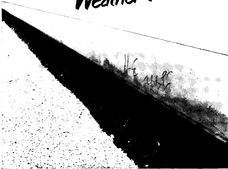
Water permeable at age 60 days! Notice loose cap flashing, faulty masonry joints, loose roofing. Indiana limestone coping with through-wall and cap flashings of copper.
