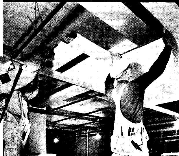
Standard 1½" Metal Channel is Used for the "Grid"
