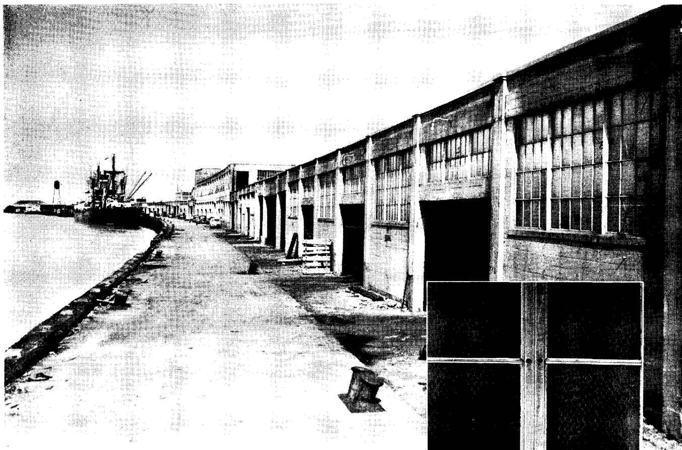
Partial view of the galvanized, unpainted Fenestra Steel Windows in the huge Mallory Pier of the Galveston Wharf Company, Galveston. And here is an unretouched closeup of one of the unblemished windows after a 23-year-long test of salt spray.
