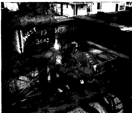
Fig. 3. Arc welding girder-to-column. This is the only weld where a scaffold was used.
