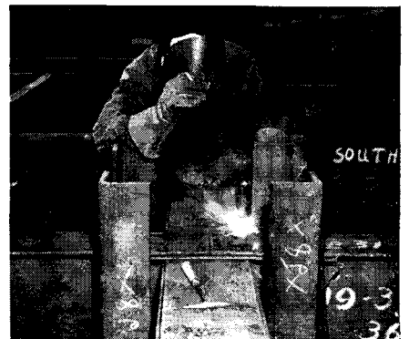
Fig. 5. Beam and girder connection made through open box column permits easy downhand welding.
