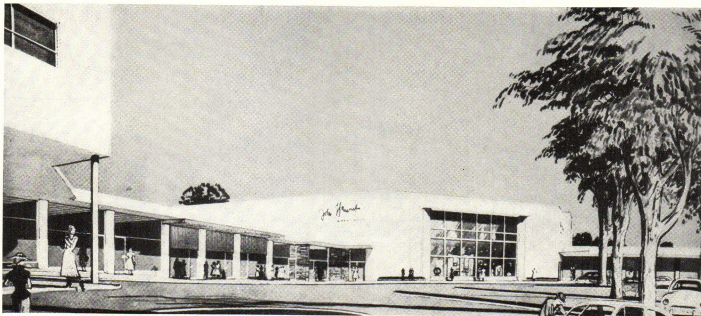
John Wanamaker Store—unit of North Shore Mart, Great Neck, New York, by Lathrop Douglass, architect, New York. Steel and concrete construction; stone ashlar and painted brick exterior walls.
