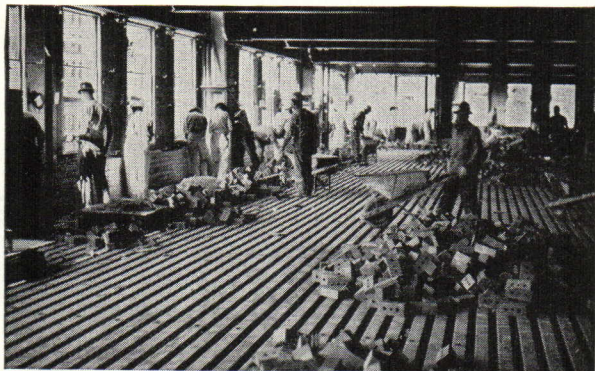
No forms or shoring to hinder them, each trade can work safely with materials and equipment immediately loaded on the Q-Floor. No need to use streets or side-walks for storage.
