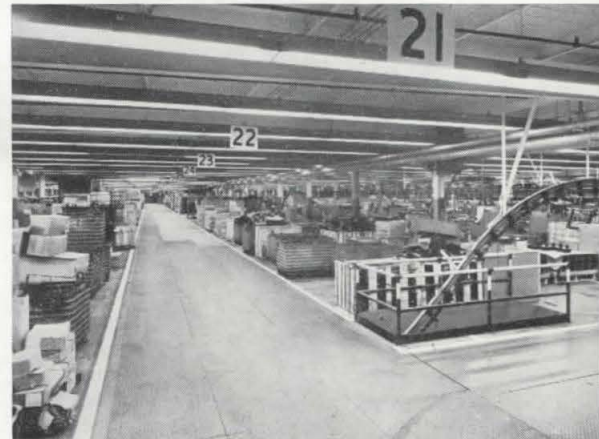
System 5, right—continuous rows delivering 50-footcandles or better are widely used in low bay areas. This installation in a large automobile assembly plant employs 2-lamp, 96" T-12 fluorescent units; on 9' spacings and 10' above floor, they deliver more than 50-footcandles.
