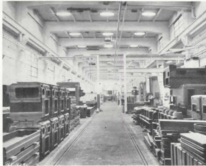
System 2, above—where maximum light per outlet is needed for high bays, 3000-watt mercury lamps offer a good solution. Each lamp emits as much light as fifty 40-watt fluorescent lamps or six 1000-watt filament lamps. Mounted 20' on center and 35' above floor, 110-footcandles are furnished. Fewer lamps require simpler maintenance.
