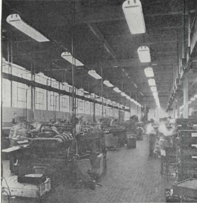
System 1, above—2 lamp, 85-watt fluorescent units in broken rows permit future expansion to continuous rows. Installed 10' on center and mounted 13' above floor, these fixtures deliver 25-30 footcandles. Walls are a light green.
