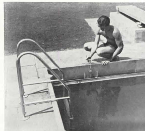
Below—adjustable overflow trough and valve permit level of water to be raised or lowered.
