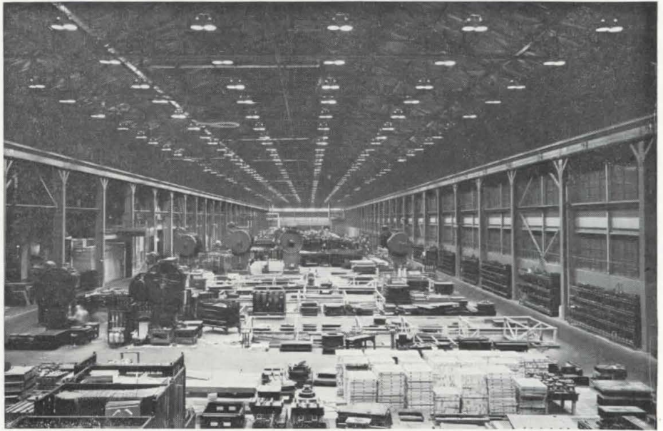
System 4, above—combination 400-watt mercury and 1000-watt filament units, mounted in pairs, 20' x 18' on center, deliver 45-footcandles. They are suitable for economical service in high bay areas where ample levels with an even blend of light are required.
