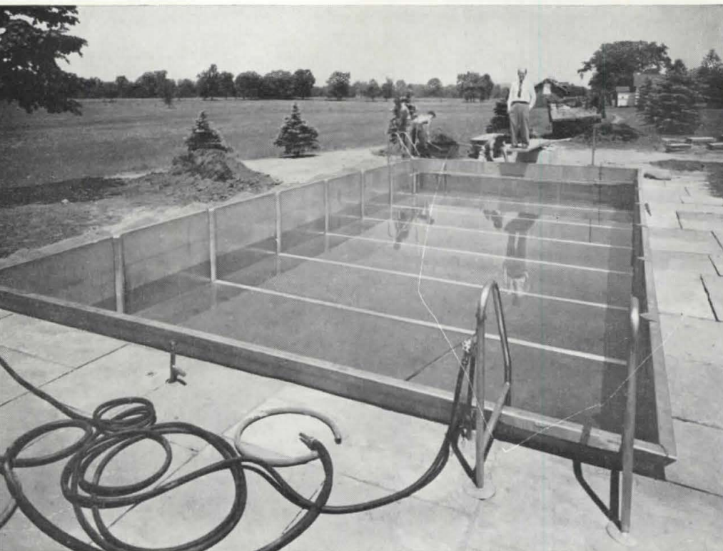
Left—sections of pool, fabricated in multiples of five feet, are bolted together; channels conceal joints.
