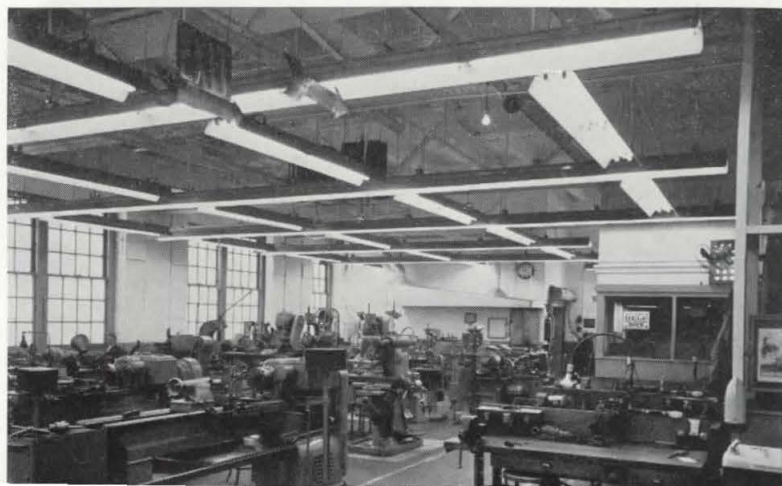
System 6, below—a grid system providing 80-footcandles from continuous rows of 2-lamp, 40-watt units.
