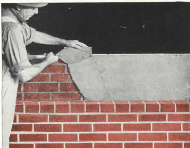
The face brick should be backplastered.
