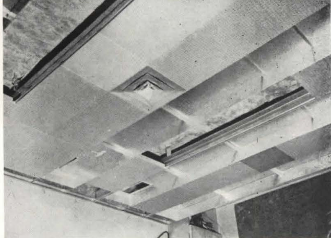
Figure 1—fluorescent troffers and the bottoms of some air ducts have not yet been placed in this partially assembled panel-cooling system.
