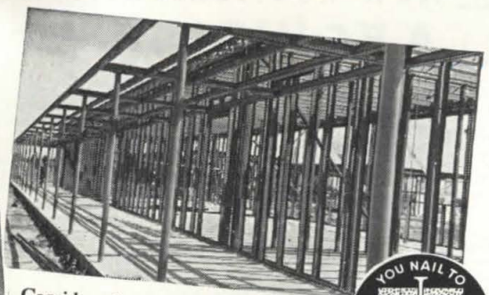
Corridor detail of school showing Stran-Steel Framing.
