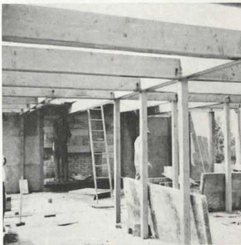
Figure 1—progress photo taken on upper level shows three 4" x 4" posts, spaced 48" on center, supporting typical roof joists; note 32" x 96" x 4" precast Cemex slab in foreground.
