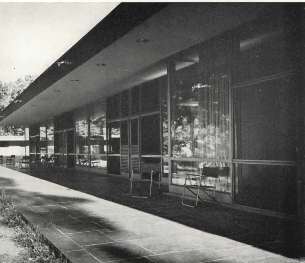
Right—the entrance terrace. Note the exposed steel frame, outside the native-stone walls; Entrance doors, in foreground, are of tempered-plate glass, in an aluminum frame.
