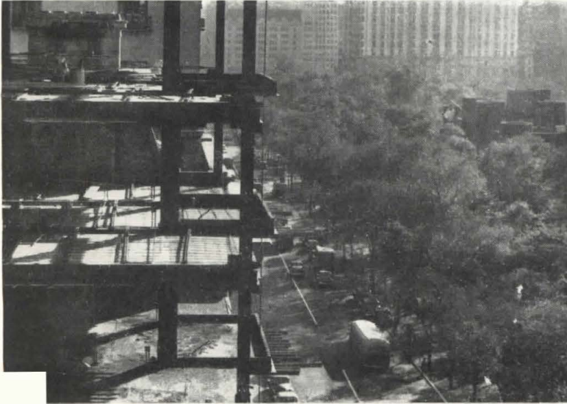
This apartment building is typical of modern steel and concrete construction. In floors, walls and ceilings, on beams, girders and columns, the continuous reinforcement of American Welded Wire Fabric keeps concrete in place, prevents cracking, helps strengthen structural members.
