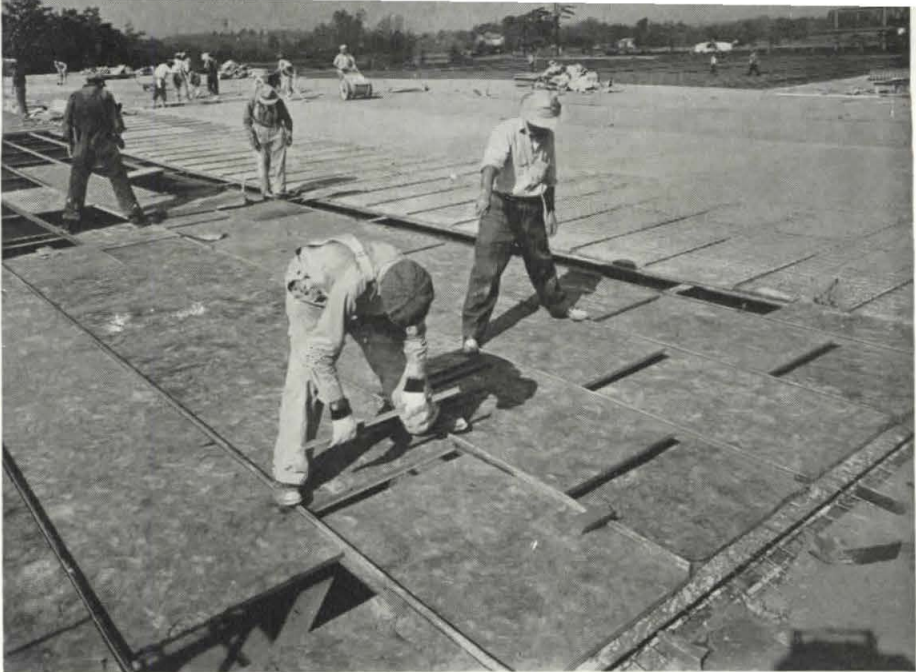
Figure 3—glass-fiber form boards in the roof of the White Laboratories plant (above) not only support poured gypsum but also provide thermal and acoustic insulation. Photo: courtesy Owens-Corning Fiberglas Corp.
