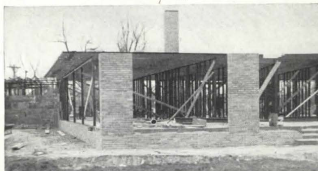
Exterior view of construction. Electrical wiring is installed through factory-punched holes in framing members.
