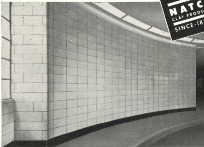
Two views showing use of Natco Ceramic Glazed Vitrile in Administration Building of the new Greater Pittsburgh Airport. View above shows long corridor lined with Natco Vitrile. View at left shows Vitrile laid in block bond construction in radial wall of main concourse. Architect, Joseph Hoover, Pittsburgh, Consultants, Parsons, Brinkerhoff, Hall & MacDonald, New York City. General Contractor, Dick Construction Company, Pittsburgh, Pa.
