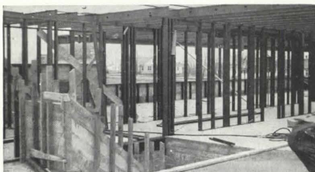
Interior view of Redfield (S.D.) hospital under construction. Stran-Steel framing comes pre-cut, pre-punched, treated with rust-inhibiting paint.
