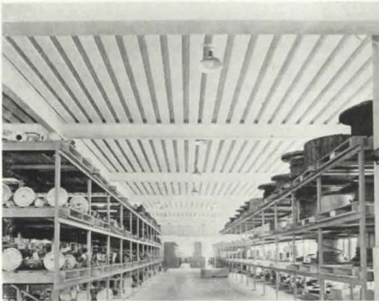
Figure 3—glass-fiber form boards in the roof of the White Laboratories plant (above) not only support poured gypsum but also provide thermal and acoustic insulation. Photo: courtesy Owens-Corning Fiberglas Corp.
