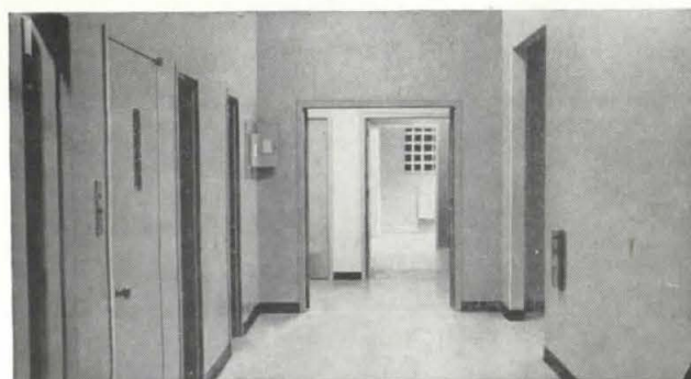
Spick-and-span interior of the hospital shows how flush finishing of walls and doors lends convenience, promotes sanitation.
