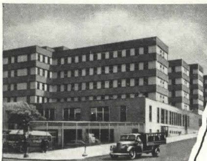
U. S. Navy residence building of Cemesto Panels and brick masonry, erected in 1939 at Brooklyn, N. Y. Contractor: White Const. Co., New York City.
