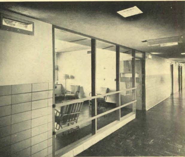
Figure 5— isolation-ward corridor looking into solarium. Two 60-watt tungsten filament lamps in each recessed louvered fixture provide an average of approximately 10 footcandles. A 15-watt filament lamp in each unit is for night lighting. Fort Hamilton VA Hospital.
