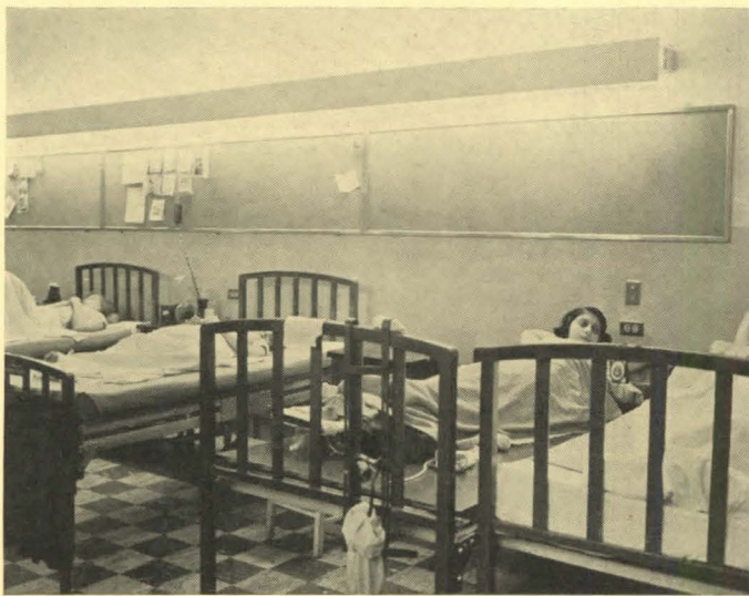
Figure 3—lighting in a children's ward. There are two rows of fluorescent lamps behind the shield above blackboard. Rainbow Hospital, Cleveland, Ohio.
