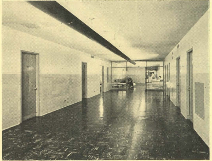
Figure 6—the corridor and reception room in the dental section are comfortably and adequately lighted to a level of 10 footcandles with two continuous rows of fluorescent lamps in an indirect fixture. Fort Hamilton VA Hospital.
