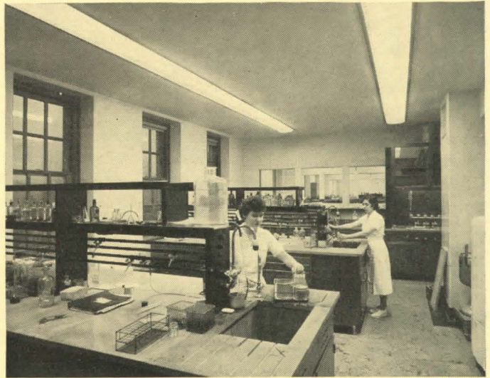
Figure 8— this chemistry laboratory is well lighted to a level of 50 footcandles. Two rows of 8' cool-white slimline-fluorescent lamps are used in each fixture. Glass coverplates diffuse the light. St. Francis Hospital, Hartford, Conn.
