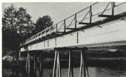
Examples of HB-construction in Sweden: Framework for a barn erected at Svalöf; span 40', height 43' (above). Decking for bridge over Viskan River at Rydal is carried on four HB-beams, continuous over piled supports; spans are 49', 66', and 49' respectively (below).
