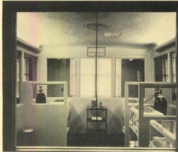
Figure 2—this premature nursery is comfortably lighted to a level of five footcandles by coves containing continuous rows of fluorescent lamps. George Washington University Hospital, Washington, D. C.
