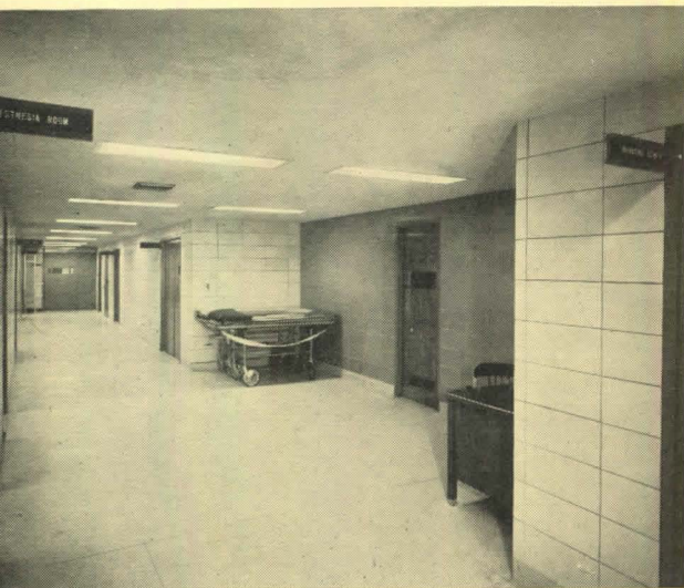
Figure 7— this surgery corridor is exceptionally well lighted, an average of 40 footcandles, with recessed fixtures containing two 40-watt fluorescent lamps. Fort Hamilton VA Hospital.
