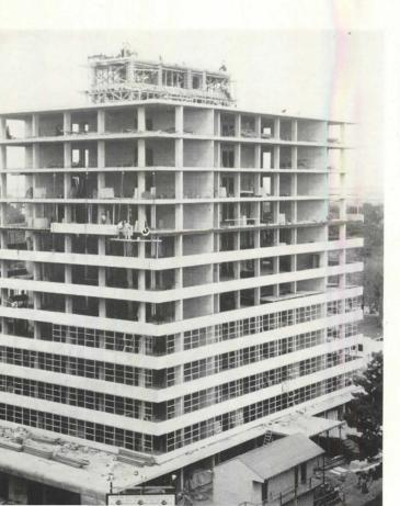
The core of the Drayton Arms, designed as a rigid frame, resists all horizontal loads and supports vertical loads. In the event of an aerial attack, the occupants would be afforded some measure of bomb-blast protection by the Photo: Andrew Bunn core.
