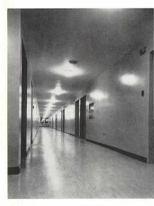
The typical nursing-unit corridor has plaster walls and ceiling, and linoleum floor. Else where, both asphalt tile and terrazzo floors are used, while the basement flooring is col ored concrete.
