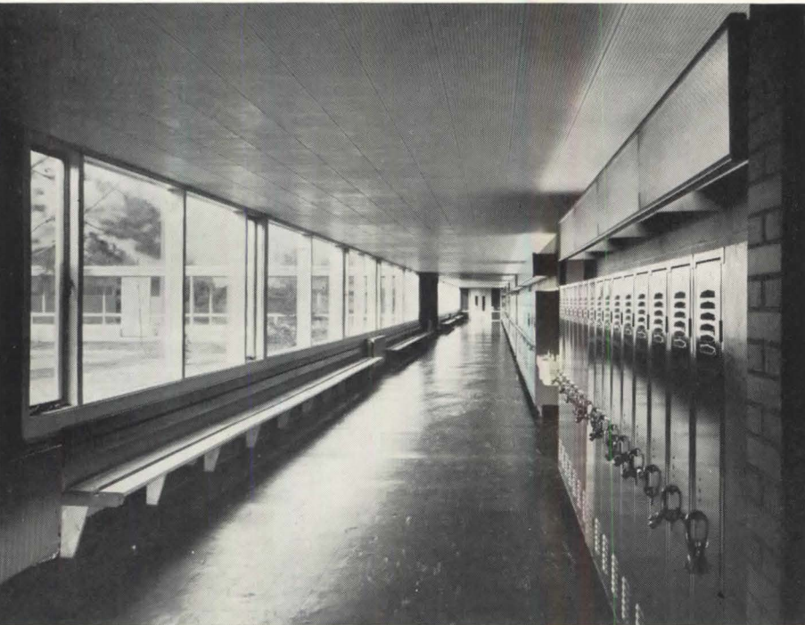
Corridors (left) and classrooms have asphalt-tile floors. Corridor ceilings are acoustic tile. Plaster is used for ceilings of classrooms, except for a strip of acoustic tile just inside the south windows. Interior walls of classrooms are painted concrete block, with acoustic-tile surfacing on upper portions.
