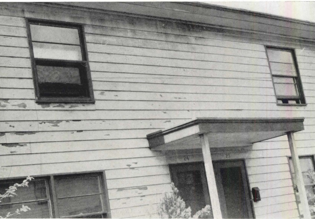
High humidity caused water condensation in the walls and ruined the paint on this apartment house (above). House siding touching the ground invites termites and decay (right).
