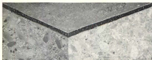
Section of Masterplate Floor. Armored Surface Approximately 1/8" Thick
