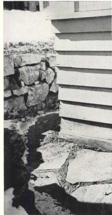
High humidity caused water condensation in the walls and ruined the paint on this apartment house (above). House siding touching the ground invites termites and decay (right).
