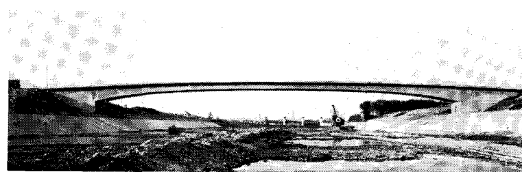
Figure 2—world's largest concrete-box girder span, across Neckar Canal near Heilbronn, Germany (above). Completed in 1950, main span of 312 ft has a 1:56 depth-to-span ratio.
