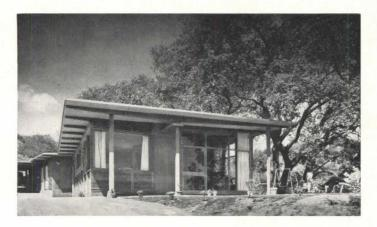
The pattern of the rafter frames, fixed glass, and louvered ventilation areas is clearly shown in the porch-end view of the completed house. The bedroom detail shows a combination of fixed glass, tilt-in wood sash, and in-opening plywood panels beneath that serve the ventilating louvers.
