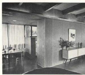
Interior wall surfaces are of striated plywood on stud frame; the cement floor is integrally colored. The house has a radiant-heating system in the floor slab. The black pattern on the floor plan indicates the vertical elements of the structural system.
