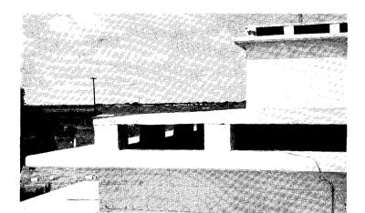
Figure 7—concrete double roof at Kano, Nigeria. Upper slab provides protection against solar radiation.
