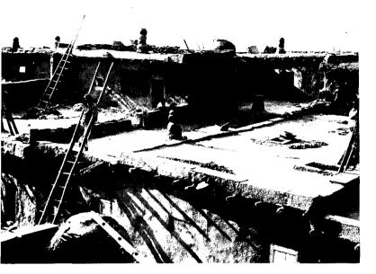
Figure 3-thick earth walls and roofs of Pueblo Indian houses in hot-dry New Mexico produced small openings and deep reveals; in addition, a longer time was required for sun heat to penetrate to the interior surfaces. *Photo: courtesy of Smithsonian Institution, Bettman Archive*
