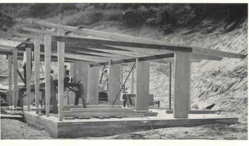
The independent structural frame (left) permits any sort of enclosure within reason. On a sloping site, the system can simply be stepped down hill (above), the roof break allowing introduction of a clerestory window. Roof edging is stainless steel.
