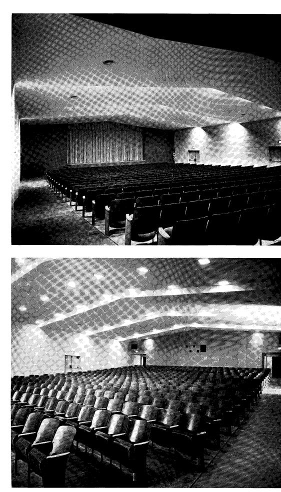
Both the walls and the ceiling of the auditorium have broken sections, which, with the semi-absorptive surfaces and glass-fiber-blanketed rear wall, provide acoustic correction. Side walls and ceiling are light gray; the front wall is dark green; and the rear wall is rose. Figuring covered area at one half, the cost of the building came to \$9.50 per sq ft.
