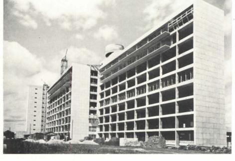
Southeast view (top), nurses' wing in foreground. Southeast approach (above) to patients' wing; plan breaks at central core, dividing floors into two nursing units. Ribbed concrete wall panels (left), cast on the site.
