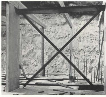
The floor slab is poured, with radiant-heating coils buried in it (above, left); note aligned steel inserts to receive framing members. The steel-channel tie member and cross bracing (above, right) occur between the interior core frames.
