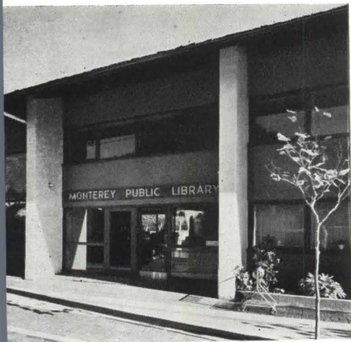
As the photographs indicate, the outdoor reading court is as yet undeveloped. The exposed concrete buttresses along the two streetfronts (left and below) effectively shield the large glass areas. A partial basement occurs under the adult reading-room wing and contains heater room and storage space. The plan shows a future additional bay and window at the end of the wing.
