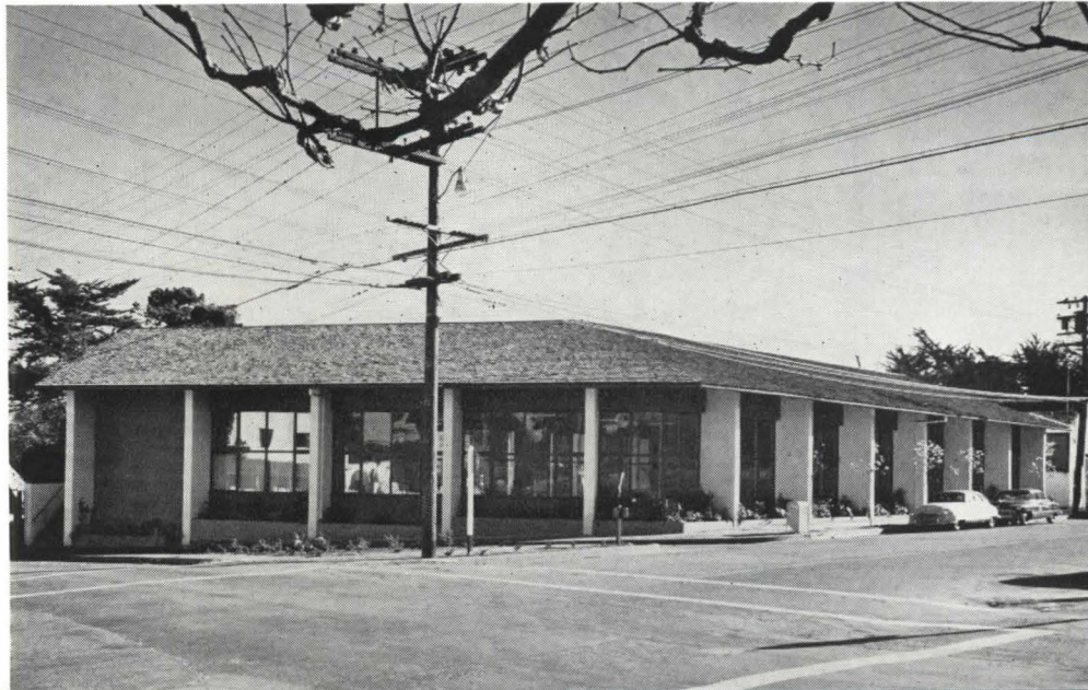
As the photographs indicate, the outdoor reading court is as yet undeveloped. The exposed concrete buttresses along the two streetfronts (left and below) effectively shield the large glass areas. A partial basement occurs under the adult reading-room wing and contains heater room and storage space. The plan shows a future additional bay and window at the end of the wing.
