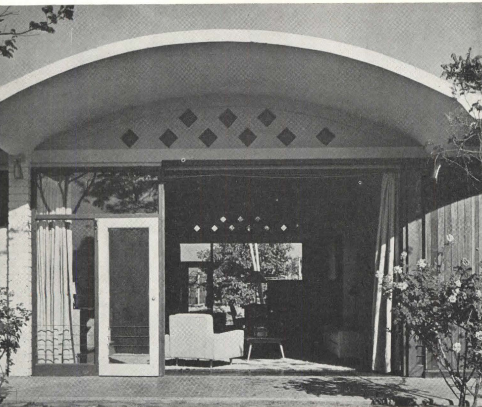
Figure 2—Fleischmann residence, Palmira (near Bogota), Colombia. Sliding-glass walls on opposite exterior walls (42 ft apart) allow complete penetration of prevailing breezes into living and dining areas of this home. The continuous barrel-vault roof projects six feet on either side of the house to afford good protection from the direct rays of the sun. J. Arango & F. Murtra: Architects-Engineers.
