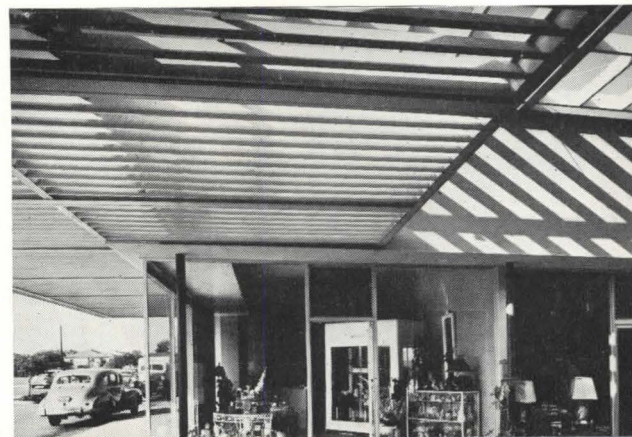
Figure 3—complete shade without sacrifice of air movement was provided by a double canopy over the arcade of the Baldwin Hills Shopping Center, Los Angeles. Robert E. Alexander: Architect.
