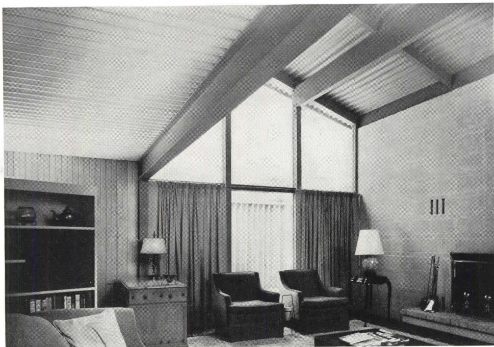
Corrugated, reinforcing-steel panels serve as forms for lightweight-concrete roof and floor slabs as well as exposed ceilings in the Hutchinson house at Glendale, Missouri; Architects: Fischer & Campbell Associates, Kirkwood, Missouri.
