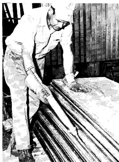
Typical panel (left) has glass-fiber insulation between stainless-steel facing and galvanized-steel back-up sheet. A 14-sq-ft panel (below left) weighing but 98 lb can be easily carried by two men. Just before erection, workman calks joint flanges (below right) as proper sealing builds up vapor barrier over entire exterior of wall to reduce "U" factor. Two men bolt panel to structural steel at sill, in freezing weather (right).
