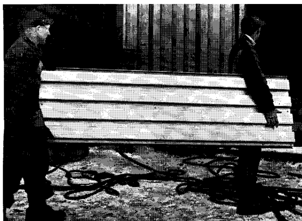
Typical panel (left) has glass-fiber insulation between stainless-steel facing and galvanized-steel back-up sheet. A 14-sq-ft panel (below left) weighing but 98 lb can be easily carried by two men. Just before erection, workman calks joint flanges (below right) as proper sealing builds up vapor barrier over entire exterior of wall to reduce "U" factor. Two men bolt panel to structural steel at sill, in freezing weather (right).
