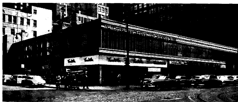
Two early examples of metal curtain-wall construction designed by Architects Holabird & Root & Burgee, Chicago. A. O. Smith, Corporation Science Building, Milwaukee, Wisconsin (left) erected in 1928 is enclosed by fixed-glass lights, held in an aluminum grillage. Monroe-Dearborn Building (right, above) 1935 is enclosed by stainless steel, backed with laminated-plastic spandrels and glass set in stainless steel.
