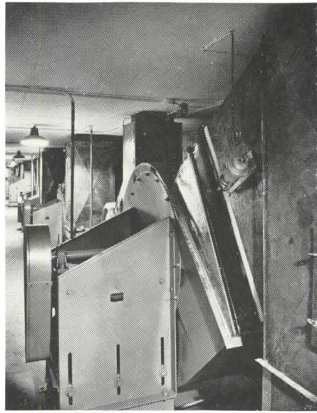
Figure 8—covered main supply duct above corridor ceiling with branch connection for exhaust grill in laboratory (right above).
