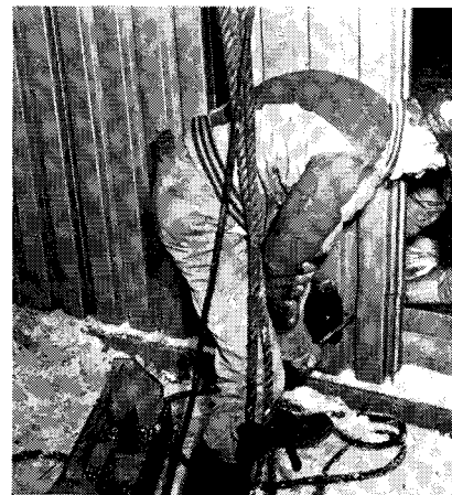
Typical panel (left) has glass-fiber insulation between stainless-steel facing and galvanized-steel back-up sheet. A 14-sq-ft panel (below left) weighing but 98 lb can be easily carried by two men. Just before erection, workman calks joint flanges (below right) as proper sealing builds up vapor barrier over entire exterior of wall to reduce "U" factor. Two men bolt panel to structural steel at sill, in freezing weather (right).
