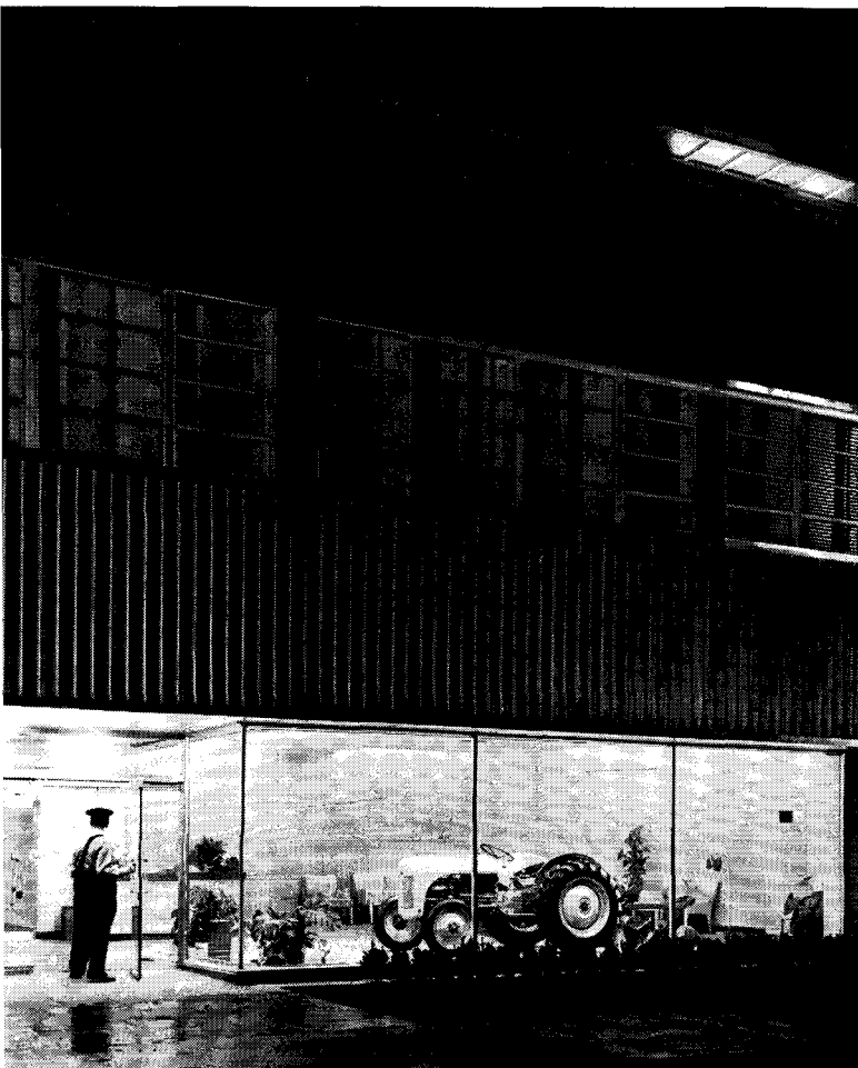
Reception room off main entrance of office building displays merchandise to be marketed (left). Each of the prefab insulated-aluminum panels on north elevation is approximately 7' high. Conference room on third floor (above) has both flush-type fluorescent lighting and down lighting.
