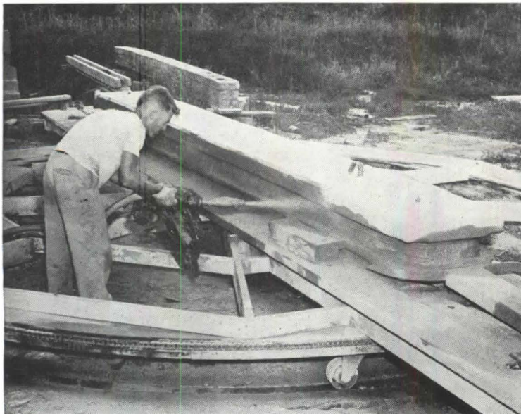
Figure 4—27' prestressed-concrete beams constructed by Preload-Crom wire winding method being placed in position (right).
