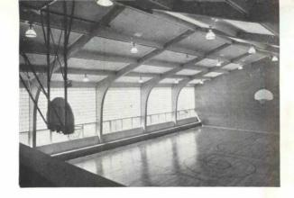
Acoustical ceiling tile between exposed roof beams handles the sound problem very well. Tinted chalkboards get strong diffused light from roof bubbles. Note how windows rise between roof beams, to the ceiling. Classroom coat rack, in front of sinks (below), can be wheeled around and used as a screen.
