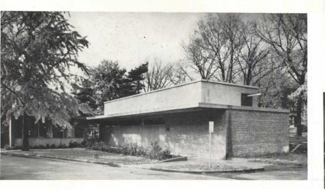
Heavy sculpture materials are brought into studio on I-beam winch track (above and below) through ceiling-height doors. Limestone, brick, and corrugated asbestos cement are used for facing materials over reinforced-concrete structure.
