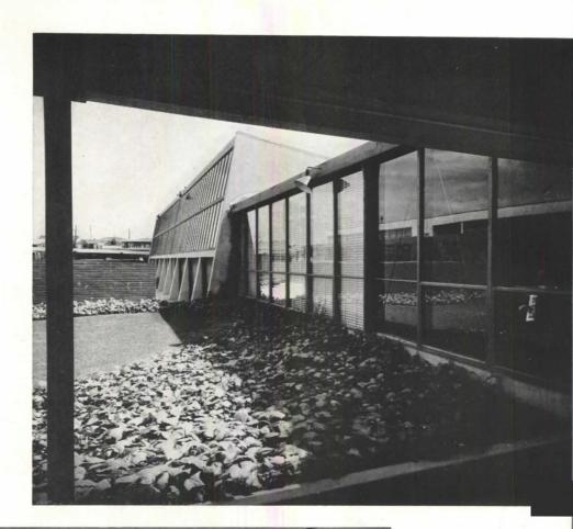
The upsloping, welded-steel bent frames of the arts and crafts building hold tall windows that provide ideal north lighting. Areas beneath consist of double doors that open the main rooms fully to the walled patio that also serves as an outdoor classroom. The low element in the foreground (right) contains teachers' rooms, toilets, and lockers.
