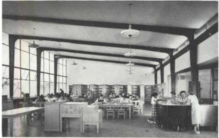
The library, with space for 10,000 volumes, is in a wing at the rear of the administration building. The bordering landscaped patio is used for outdoor reading. Framed in welded-steel bents, the building has ceiling-height windows along the north wall; a narrow, louvered window band occurs at the ceiling line on the south wall.
