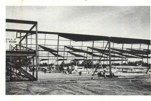
Designed to support a total load of 22 psf (12 live/ 10 dead), each tapered-steel girder has the following dimensions: length, 60'; mid-span depth, 42"; depth at ends, 16"; flange width, 10"; flange thickness, 3/8"; web thickness, 1/4"; weight of girder, 3000 lb (1.7 psf average). All 36 tapered-steel girders required for the machine shop are supported by 6 WF 15.5 columns.
