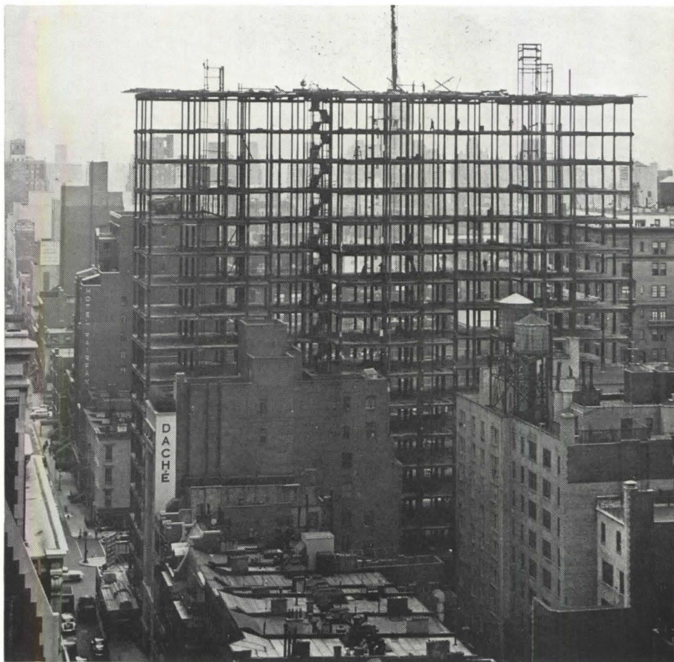
All that remained of original apartment house after demolition were its framework (columns are shown in black, acrosspage), concrete floor arches, and foundations. New work is shown (in black, below).
