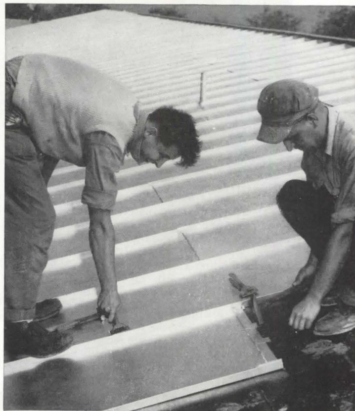
INSTALLING the standing-seam USS Stainless Steel roof on the new Walnut Grove School. The roof was laid on double-coated asbestos felt with each cross seam carefully caulked before the upper sheet was installed.
