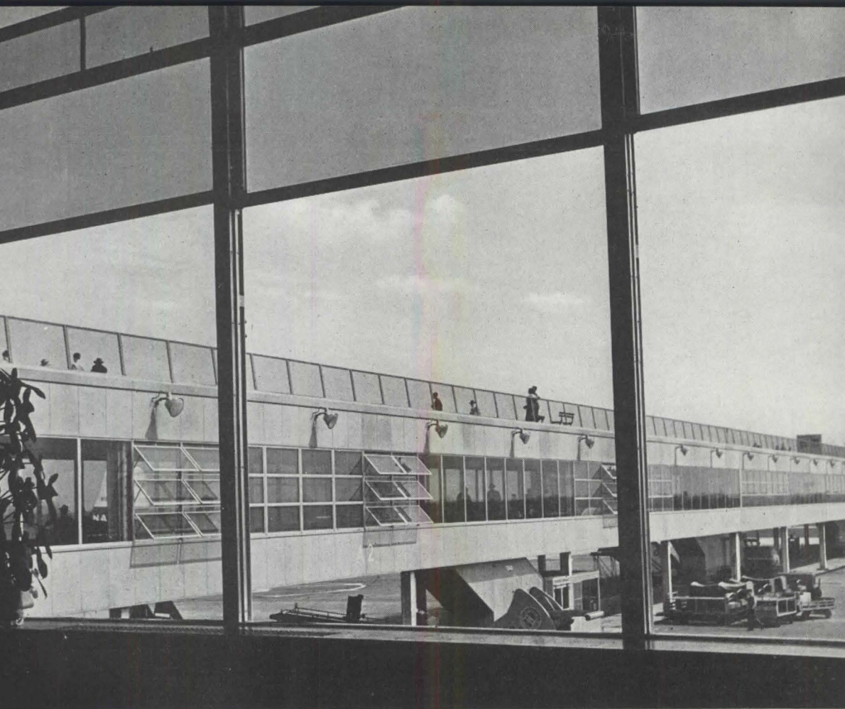
The two finger concourses extend some 500 ft onto the field and are bordered by plane stations. Roof of the finger on the east (above) is used as a visitors' observation deck (admission: 10 cents). The open ground-floor level speeds the movement of baggage and other services; from the passengers' enclosed second-floor level (right), stairways lead down to the field. When expansion is necessary two more fingers are planned—one at the east end of the terminal; the other on the west.
