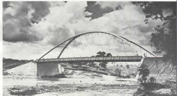
Labored abutments detract from clean pattern of steel in this structure over Cape Cod Canal (above left).
