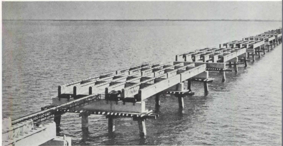
Bridges in Florida (above) and Venezuela (bottom of page) show possibilities of prestressed concrete in overcoming difficult erection problems.
