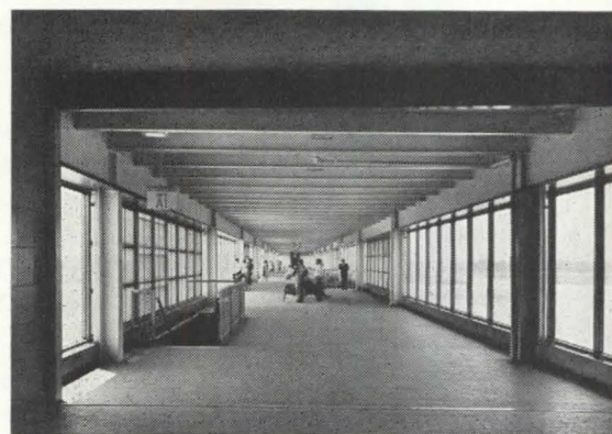
The two finger concourses extend some 500 ft onto the field and are bordered by plane stations. Roof of the finger on the east (above) is used as a visitors' observation deck (admission: 10 cents). The open ground-floor level speeds the movement of baggage and other services; from the passengers' enclosed second-floor level (right), stairways lead down to the field. When expansion is necessary two more fingers are planned—one at the east end of the terminal; the other on the west.
