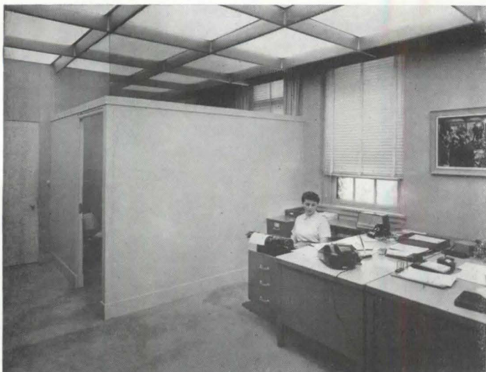
Figures 2 and 3—a new form of luminous ceiling employs arched sheets of acrylic plastic in metal frames resting on criss-crossed bars of perforated metal with glass-fiber packing for acoustic treatment (below). Metal frames are hinged and drop open to permit access to lamps and easy cleaning of plastic (below right).
