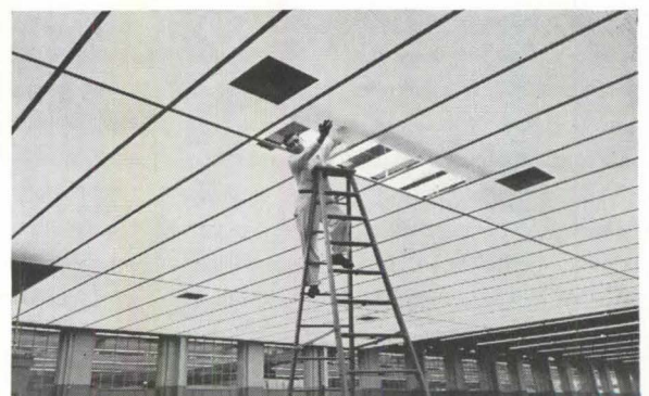
Figure 8—workman completes luminous ceiling installation above drafting tables in the Engineering Administration Building of the Ford Motor Company, Dearborn, Mich. (above). Continuous slim-line fluorescent light sources are hung above corrugated plastic. Diffusers slide back to expose lighting units for service.
