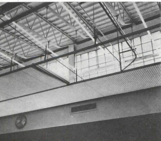
Figure 4—glass-block panel above luminous ceiling in classroom contributes daylight; Architects—Sargent, Webster, Crenshaw & Folley. Lightweight corrugated-vinyl-ceiling is rolled back for maintenance (left).
