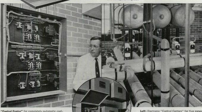
"Control Center" for completely automatic cooling, heating, rehumidification, reheating systems. Serves as central junction box, houses prewired ac-
