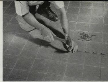
Hardboard or plywood underlayment should be firmly nailed to the underfloor with coated or ferrule-ring nails. Nails must be placed not over six inches on center in all directions and at all edges and driven flush with the underlayment.
