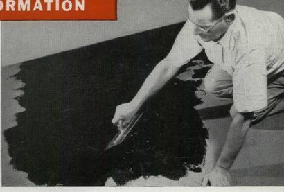
Armstrong No. S-105 Chemical-Set Underlayment Cement may be troweled to a thin "featheredge" in leveling worn or damaged areas of concrete subfloors. This will frequently eliminate the need for complete resurfacing of an old subfloor.
