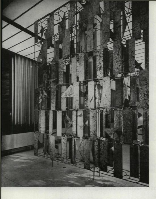
Bertoia used an acetylene torch to cut the steel accent motive (below) and the plaques, as well as for melting brass, nickel, and copper to flow over the plaques. The screen was lacquered, for preservation, and is dramatically illuminated by spotlights.
