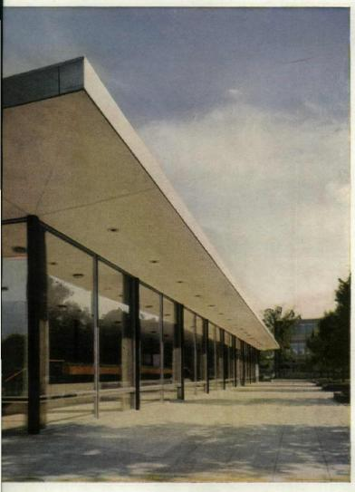
The building has a metal-deck roof with wide overhang. Detail of window wall (top right) at west elevation, makes a handsome composition of metal louvers, porcelain-faced insulated panels, and glass set into extruded-aluminum frames within the structural steel module, spaced 18' on centers.
