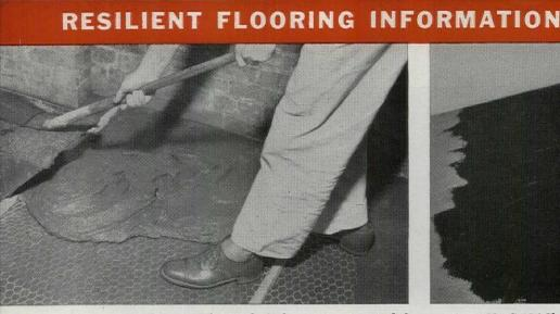
Over wood subfloors, galvanized chicken wire or expanded metal lath should be nailed to the floor to reinforce cold mastic floor fill. The wire netting allows the wood floor to expand and contract without cracking or damaging the floor fill.
