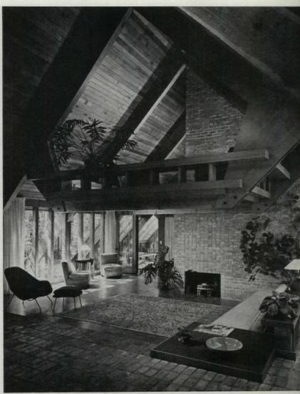
The giant rafters extend beyond the envelope to supporting concrete buttresses. To skylight the gallery and screened porch, portions of the roof are glazed. Floorings are either brick or cork, and the house is heated by a radiant system, employing copper coils.
