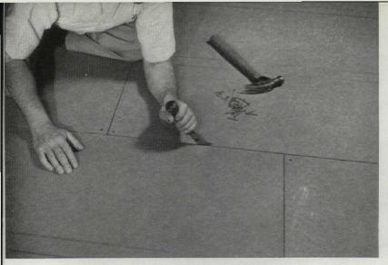
Joint spacing of approximately 1/16" is left between sheets of hardboard underlayment to allow for slight expansion and contraction with varying moisture conditions. The hardboard sheets should be laid with joints staggered, ashlar fashion.
