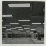
Connected lighting load, approximately 450 KW. Maintained lighting level, main thoroughfares, 22 foot-candles. Maintained lighting levels, distribution center, 30 foot-candles. Average parking area illumination, 10 foot-candles.
