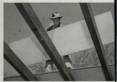
1. It's roof deck . . . Two by eight foot unit cuts application time as much as 45%. Only one material to handle. New Insulite Roof Deck eliminates need for separate roof boards, insulation, lath and plaster and ceiling finishing. Roof Deck can save 12 man-hours per 1,000 sq. ft. of surface compared with 2"x6" D&M roof sheathing.
