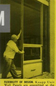
FLEXIBILITY OF DESIGN. Knapp Unit Wall Panels are assembled at the factory with the exception of glass. Each unit is complete with insulated metal panels and ventilator completely caulked. They provide full flexibility of design. Ventilators, fixed glass and insulated panels can be varied to meet the individual requirements of the job.
