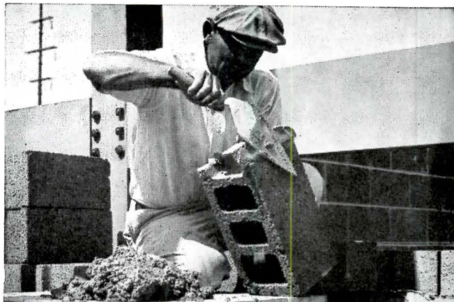
EXCEPTIONAL WORKABILITY — Contractor Frank Scheck, working on Oswalt Company's concrete block plant at Broadview, Ill., says, "Atlas Mortar holds its plasticity... does a better job—faster."
