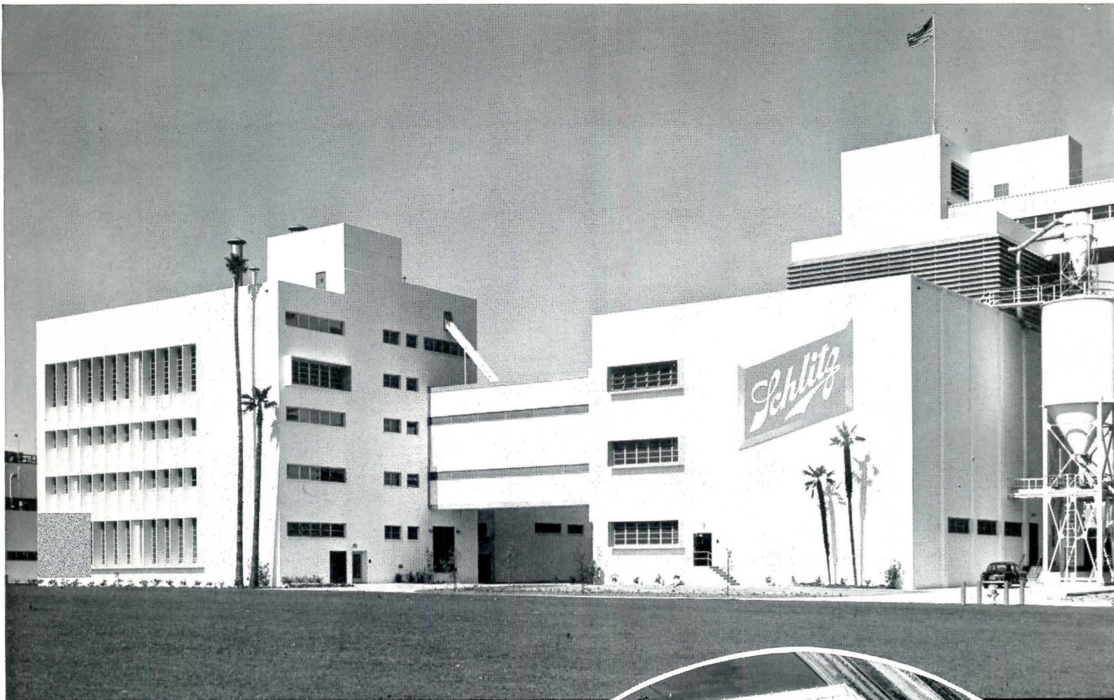
Schlitz Brewing Company, Van Nuys, California Archts.—Harley, Ellington & Day, Detroit Consltg. Struct. Engrs.—Brandow & Johnston, Los Angeles Gen. Contr.—P. J. Walker Co., Los Angeles Pozzolith Ready-Mixed Concrete supplied by Arrow Rock Co., Sun Valley, California
