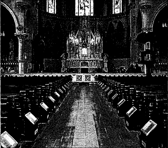
Carrier Fan-coil Units are located around perimeter walls and at pew ends along center aisles in The Cathedral of the Sacred Heart, Dallas. This unique air distribution method made it possible to cut size of the air conditioning system from 125 to 83 tons.
