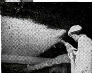
Scratch coat of plaster machine-applied direct to metal lath.
