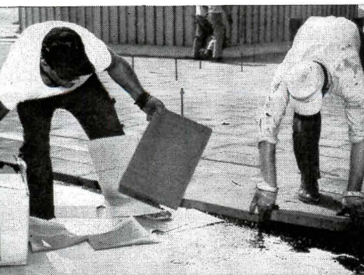
"We also insulated most roofs with FOAMGLAS. Its high strength permits heavy foot traffic, minimizing need for catwalks.
