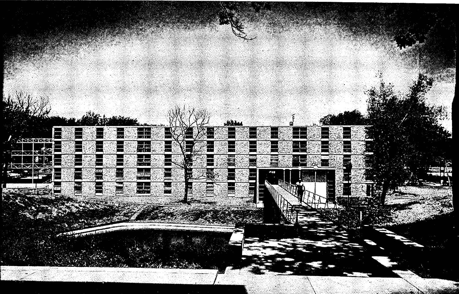
Dormitory #1 (below), seen from restaurant, has direct bridge connection with balcony of social room. Regular grid pattern of dormitory building is a clear expression of the tilt-up slab construction employed.
