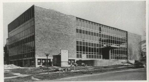
NIAGARA COUNTY BUILDING, NIAGARA FALLS, N. Y. Arch: Charles F. Obenhack. Contr: Walter S. Johnson Building Co. Lupton Curtain-Wall System, Type G. Width module, 4'-0". Double glazing, 1" thick fixed lights, ½" thick in ventilators. Ventilators open in. Opaque areas are double panel construction. Outside face is greenblack porcelain enamel laminated with honeycomb core, galvanized back. Inside face is galvanized steel sheet covering 1" thick insulation. Back-up wall to sill height.
