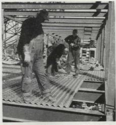
Cofar for Concourse Floors. Webb-Winn-Senter speeded the casting of concrete floors by using Cofar which acts as a deck for workmen, a form for wet concrete, and as reinforcing when the slab sets.
