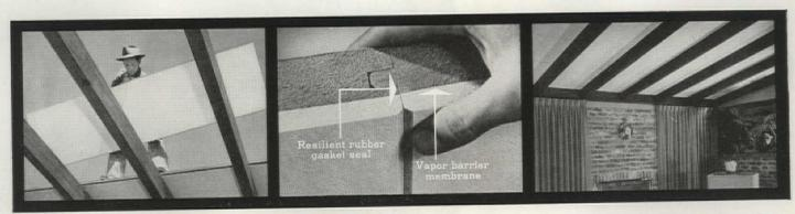
1. It's roof deck . . . Two by eight foot unit cuts application time as much as 45%. Only one material to handle. New Insulite Roof Deck eliminates need for separate roof boards, insulation, lath and plaster and ceiling finishing. Roof Deck can save 12 man-hours per 1,000 sq. ft. of surface compared with 2"x6" D&M roof sheathing.
