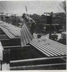
Granco Steel Roof Deck formed concourse roof and decorative curtain wall behind upper-deck rear seats. Wide sheets meant fewer laps, greater roof strength and safety, time saved in placing and welding.
