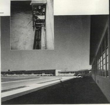
MICHIGAN. Long, low and handsome. Edmonson Elementary and Junior High School, Willow Run, Mich. Installation cost of Herman Nelson DRAFT STOP System was materially reduced by laying piping on depressed slab in exposed perimeter trench (see inset), with unit ventilators and utility cabinets serving as cover. Superintendent of Schools: Albert C. Johnsen; Business Manager: A. A. Wiench; Architect and Engineer: W. T. Anicka; Mechanical Contractor: United Heat Engineering Co.
