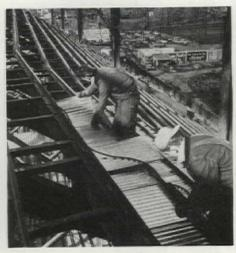
Corruform between Risers. The 100,000 psi steel made both concrete base and working platform, kept laying crews well ahead of concreting. Hot-dip galvanized Corruform was vinyl primed for painting.
