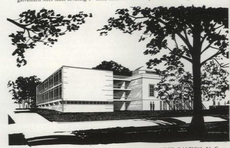
SCHOOL OF DESIGN, NORTH CAROLINA STATE COLLEGE, RALEIGH, N. C Arch: F. Carter Williams. Contr: Dickerson, Inc. Lupton Curtain-Wall System, Type H. Width module, 5'-8". Fixed glass and ventilators are inside bead glazed. Ventilators open out. Spandrels and column faces are covered by aluminum sheet .102" thick,
