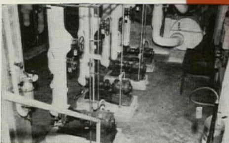
Installation of B & G Universal Pumps for circulating heating and cooling circuits.
