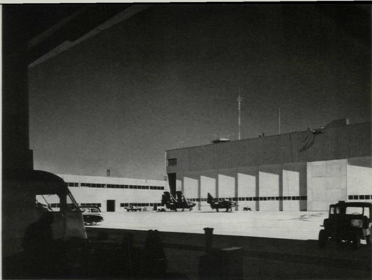
Two leaves of each of the 140-ft-wide hangar doors contain a pass door, and all leaves have glazing above eye level. To prevent freezing in winter, steam pipes are provided under the tracks of the doors. The doors are painted a brilliant yellow.
