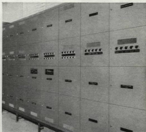
Modern "Control Center" (above) in remodeled building serves as central junction box, houses prewired accessories, numbered terminal strips, indicating lights, remote starting buttons, etc. A Uni-Flo "VF" Grille provides ventilation of each compartment.
