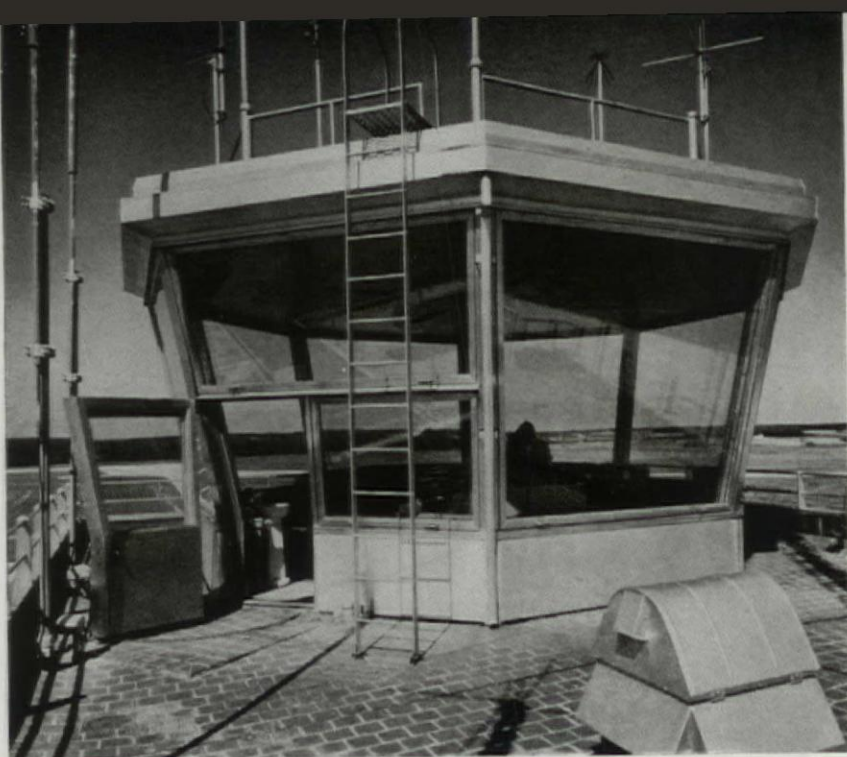
The control room is exceptionally well insulated for obvious reasons—acoustically treated; double glazing, separated by a 4-in. air space (outer pane, of heat-absorbing glass); acoustic pan ceiling; and heavy carpeting. Roof is of stainless steel to reflect heat; and stainless steel mullions were used to minimize obstruction to view.
