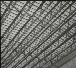
ABOVE: Used as a form for short-span concrete slabs, % in. Milcor Stay-Rib No. 2 provides rigidity and does not depend on being stretched taut to carry wet concrete. BELOW: Underneath view shows how slab and steel joists are bonded together in a rigid floor system.
