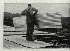
Handles Easily, Places Fast. Tufcor arrives pre-cut to building size. Measuring and cutting is eliminated. Two or three men can place up to 10,000 sq. ft. a day.
