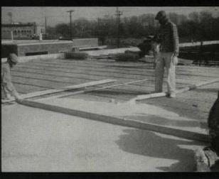
Typical installation of new PYROFORM Formboard, on steel cross tees. New process felts and bonds mineral fiber into boards, 1" x 32" x 48". T. M. Reg. U. S. Pat. Off. Pouring PYROFILL slurry. Outstanding advantages: incombustible, low in cost, adaptable, light-weight, strong, durable, quickly installed.
