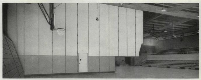
**Brunswick-Horn** Folding Partitions convert one gym into two in a matter of minutes . . . lock quick and quiet without bolts . . . automatically seal with floor.
