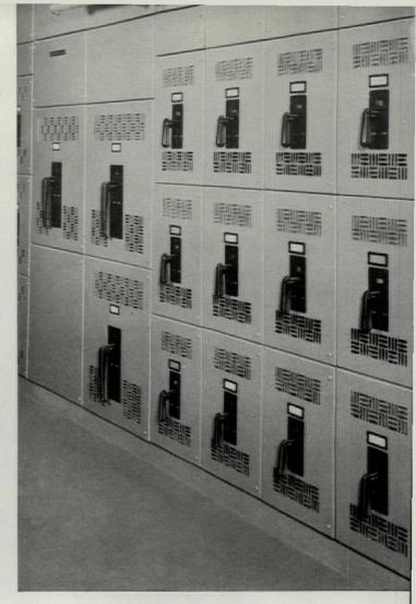
**Building-type switchboard** is a factory-assembled unit containing modern circuit breaker protective devices. Switchboard is compact and completely safe.
