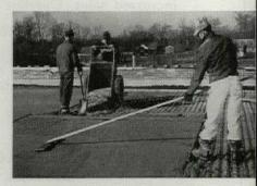
Permanent, Fire-Resistant Roof Deck is formed by cast-in-place slab. A strong bond forms between galvanized steel sheet and lightweight concrete fill giving high-strength rigidity to finished deck.
