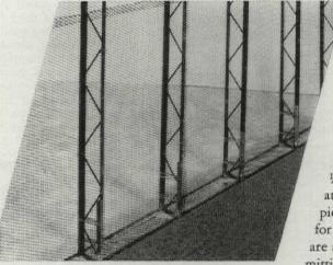
Gold Bond Holostuds can be put up simply and quickly. All connections are made easily with wire ties. Ordinary lather's tools are all that is required to erect the entire Holostud Wall System.
