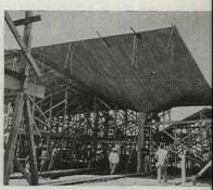
Thickness of each umbrella slab is only  $1\frac{1}{2}$  in. Formwork for individual tympan is dropped separately and moved to next pouring position (above).
