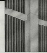
DETAIL OF SPANDREL, MULLION AND PILASTER
