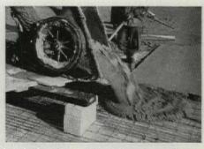
**Insulating Concrete Placed on Tufcor** is fast operation. On an average roof construction, this material weighs less than 6 pounds per square foot.
