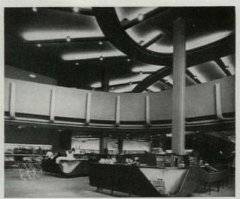
Kline's West, Carrier-equipped department store in St. Louis, has a unique air duct system. Conditioned air comes from "trees"—ceiling-suspended, tree-like lighting troughs centrally located over main floor and mezzanine.
