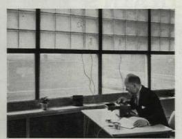
Thermocouples applied to the face of the 80-F block during hot weather (outside temperature  $90^{\circ}$ ) showed that the roomside surface temperature was 14 degrees less than a conventional type light-directing block.
