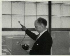
A similar test using a portable pyrometer confirmed the findings of the test using thermocouples by showing the same 14 degrees lower temperature on the roomside surface of the 80-F glass block.
