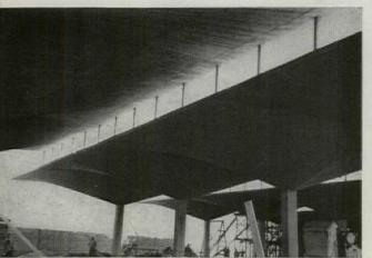
By tilting umbrellas slightly, Candela obtains a northlight, saw-tooth roof in an extremely economical manner. In a more recent warehouse of this type, he has placed glass blocks in the slabs for additional toplighting. A 6-in. asbestos-cement drain pipe is located in the core of each column. Photos: Antonio Candela
