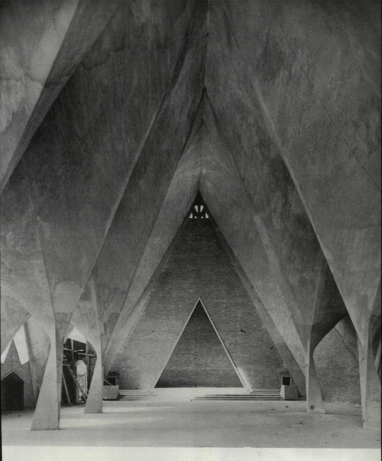
Size of typical bay in nave is approximately  $40' \ge 22'$ , width of side aisles is about 13', and vault springers are located 10' above floor level.
