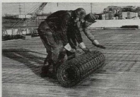
An Immediate Safe Working Deck is obtained as soon as Tufcor is attached. Light mesh is added for shrinkage control of the lightweight insulating concrete.
