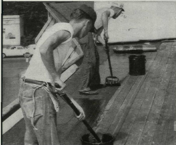
Perma-Topp being applied over wood deck after removal of old roofing. The 1st ply has been applied and 2nd ply is being started.
