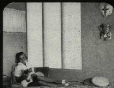
350 sq. ft. of translucent reinforced plastic panels, recessed in deep studs to block sun's glare, flood guest house with soft, shadowless light.
