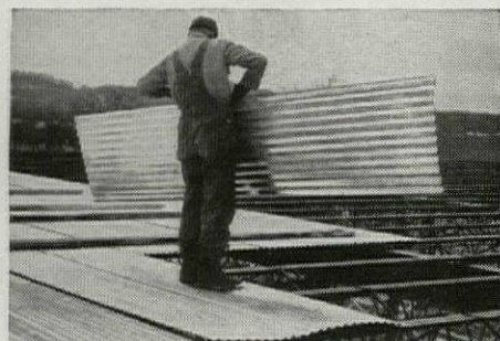
Handles Easily, Places Fast. Tufcor arrives pre-cut to building size. Measuring and cutting is eliminated. Two or three men can place up to 10,000 sq. ft. a day.
