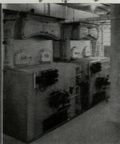
Two No. 588, 125 lb. Kewanee Boilers installed in the Hospital San Carlos in Bogotá, Colombia. They assure power expansion when needed—an important factor when the lives of patients are at stake.
