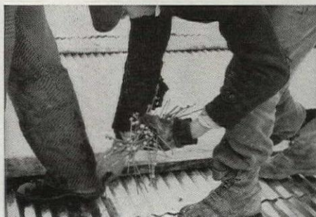
Steel Sheets Are Quickly Clipped to the steel framing. Welding is equally fast. Positive attachment of tough-temper sheets adds rigidity to roof framework.
