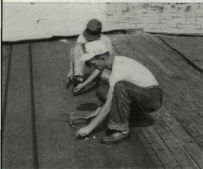
Here, the 2nd ply is being completed.
