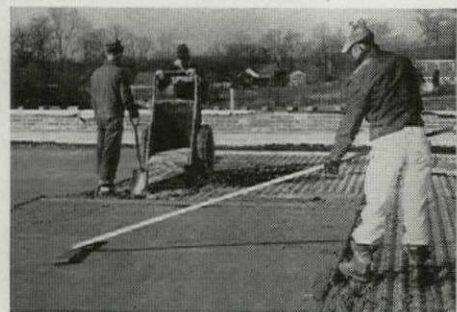
Permanent, Fire-Resistant Roof Deck is formed by cast-in-place slab. A strong bond forms between galvanized steel sheet and lightweight concrete fill giving high-strength rigidity to finished deck.
