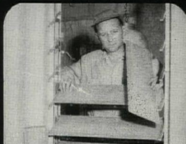
Jalousies made of low-cost reinforced plastic panels are easy to install, offer long-lasting light-ventilation control with minimum maintenance.
