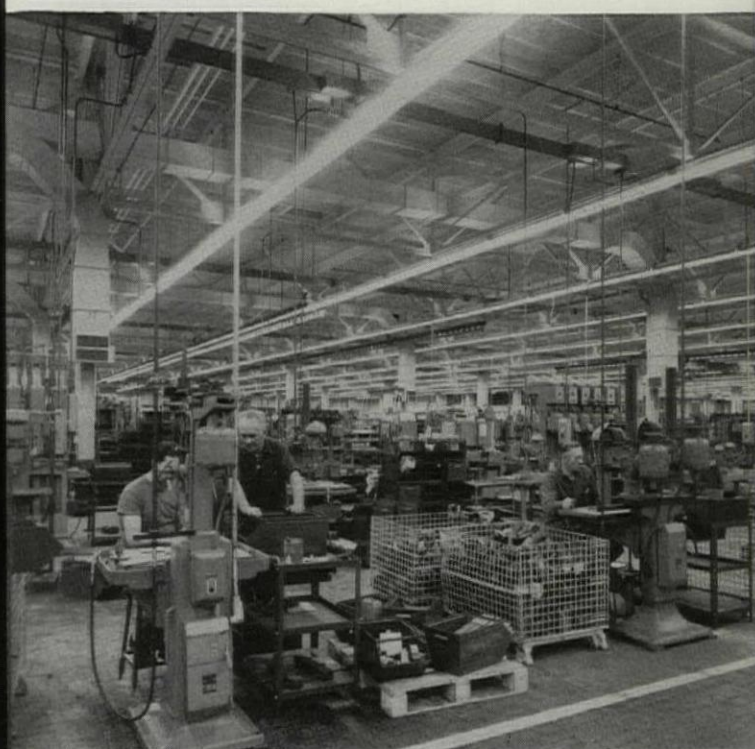
Day-Brite CFI-10 (Comfort For Industry) with 10% upward lighting. Ceiling contrasts are washed out and greater visual comfort assured.
