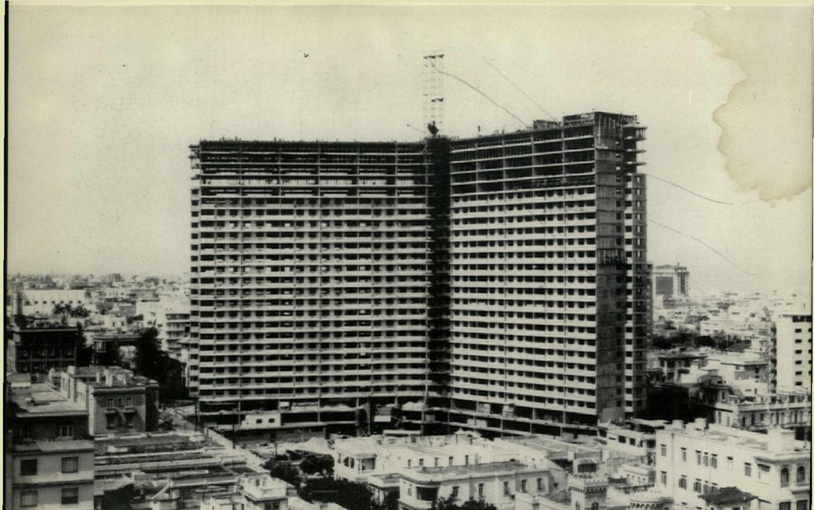
"17 y M"—Reinforced concrete apartment building, Havana, Cuba. Designed to withstand hurricane-force winds. Architect: Ernesto Gomez Sampera and Martin Dominguez; Structural Engineer: Saenz-Cancio-Martin; In charge of Construction: Bartolome Bestard and Manuel Padron.
