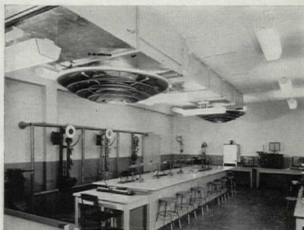
Figure 4—Exhaust hood for removal of fumes from a lead-melting pot (left). This is one example of local exhaust ventilation in industry.
