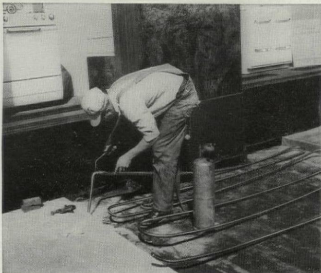
Leak-free joints made easily with torch and solder.
