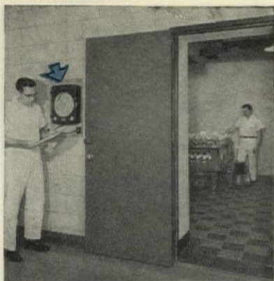
Shaker room and incubator in Fermentation Department. Powers Temperature Recording Controllers are used here.
