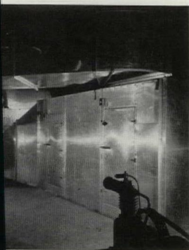
Figure 2—Central-type conditioning apparatus for maintaining desired temperature and humidity conditions (left).
