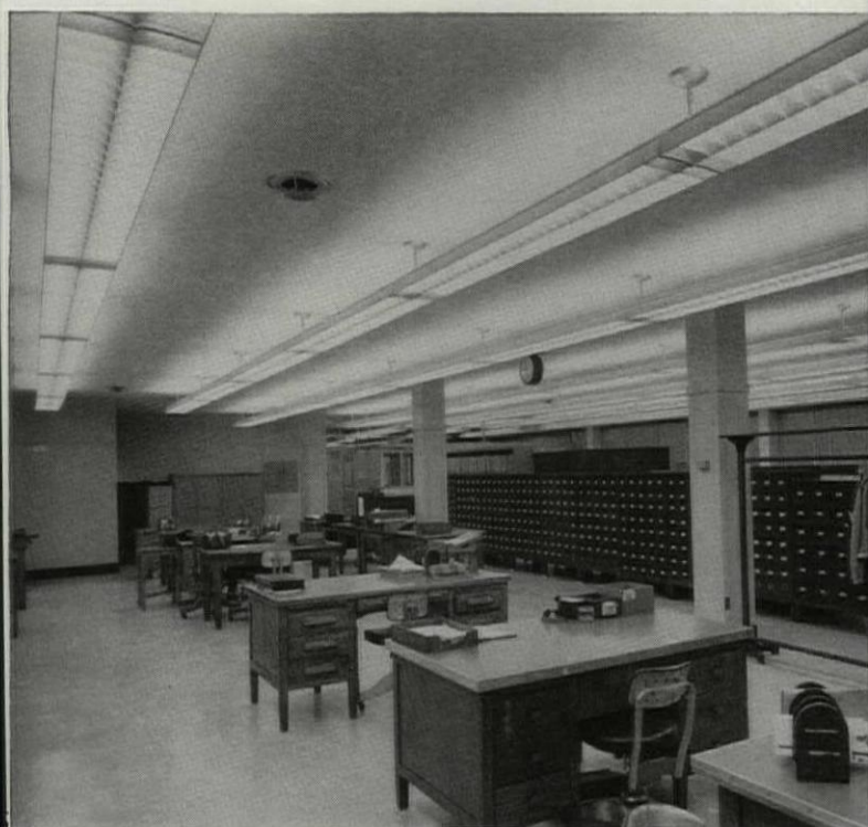
Day-Brite continuous Luvex® light this office area. Note straight-line runs and high desk-top visibility.
