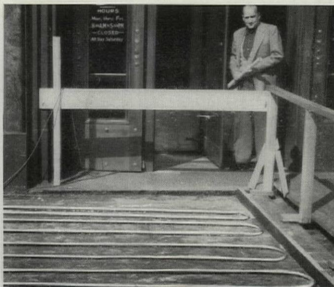
Section of system ready for paving.
