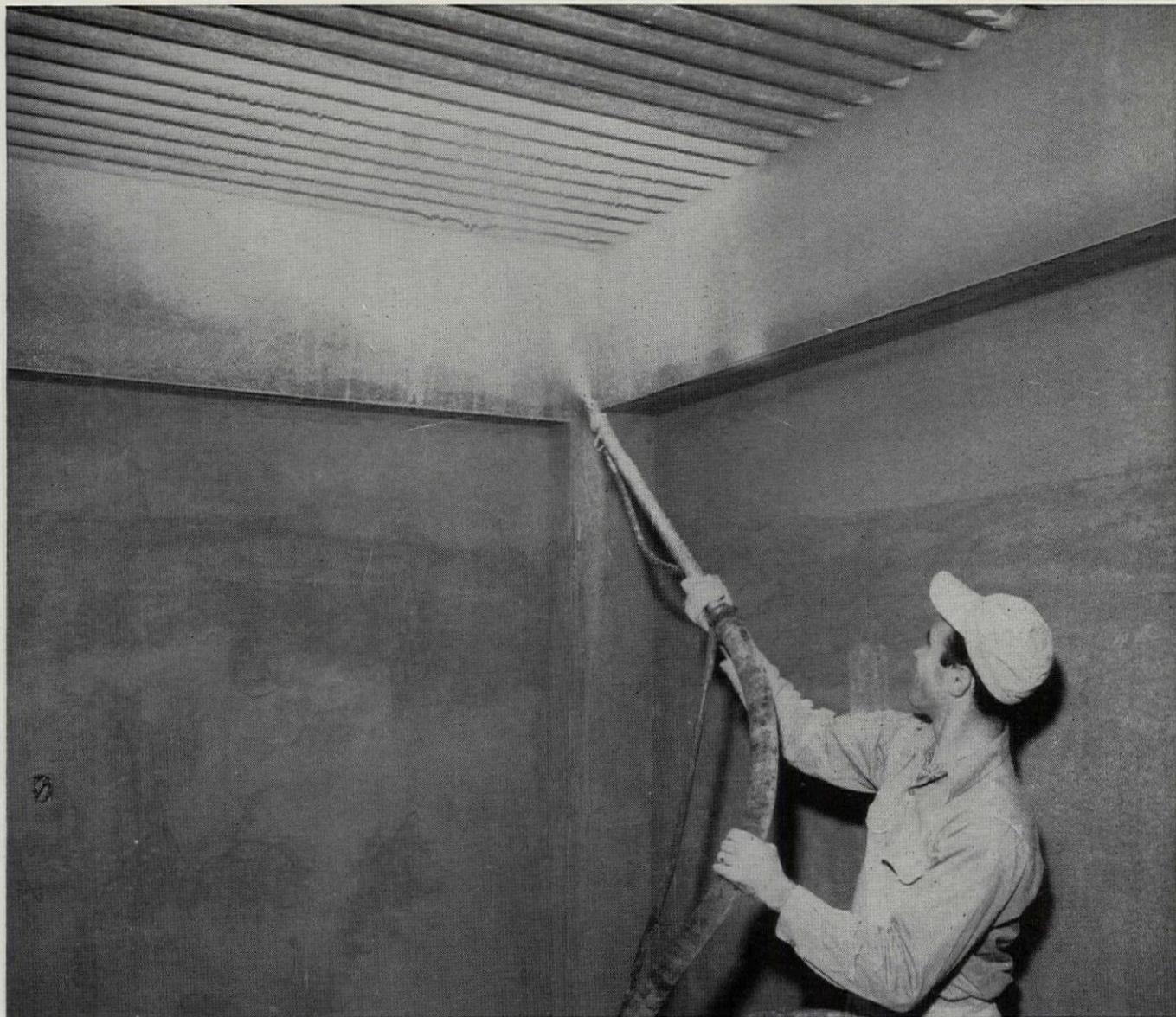
**Only 18 Days From Start to Finish!** Averaging 3000 sq. ft. per day, workmen spraying 3 coats of acoustical plastic on Cofar completed each floor in only 3 days—the entire job in 18 days!
