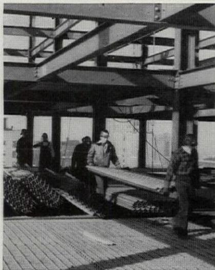
**Wood forms eliminated**—Because Cofar eliminates bulky, expensive wood forms, limited storage space on the job site was used to maximum advantage. Once installed, Cofar forms a solid, safe, sheltered working deck for all trades.
