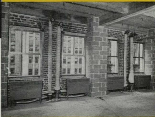
Photograph taken during construction of Seaman's Bank for Savings showing installation of Tuttle & Bailey Type MPW Double Duct Mixing Plenum Wall Units.
