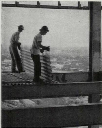
**Handles easily, places fast**—Cofar units arrived at the job site conveniently bundled and identified for immediate placing. In 8 days, 5 workmen had placed and welded Cofar into position—ready for concrete pours several days ahead of ordinary forms.
