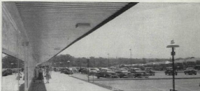
For supermarkets and schools much greater latitude of design is allowed by increasing deck span. Considerable saving in structural steel is made possible, and time and labor are cut down in the erection of the deck itself.
