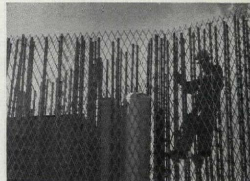
Wall area using a combination of STEELCRETE and bars to obtain desired reinforcements. Produced in 3" x 8" diamond shape, STEELCRETE offers up to 1½ sq. in. of area to the foot of width.
