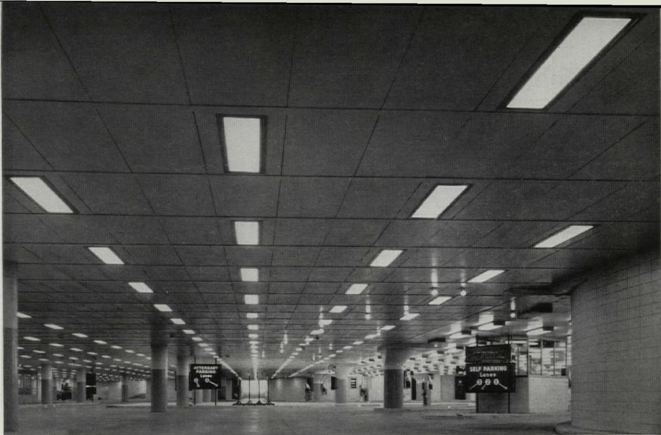
Chicago's Grant Park Underground Garage uses Corning flat and bent Alba-Lite lightingware. Alba-Lite comes in a variety of bends to provide design flexibility. Flat Alba-Lite panels are available in three patterns offering true light source transmission, exceptional brightness control by diffusion, high fixture efficiency, permanence and low upkeep cost.
