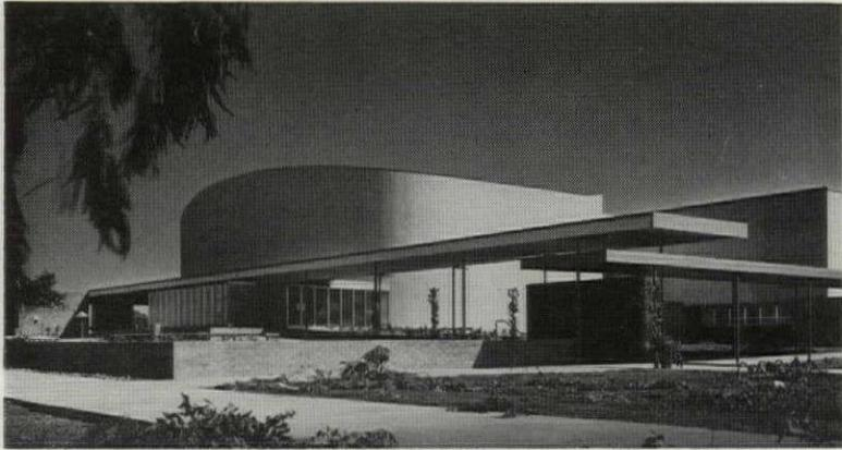
*Vertical marks on concrete walls of auditorium (left) are the result of slip-forms moved upward during construction. Rectangular structure in background encloses stage house, stage-craft facilities, heater and boiler rooms. Covered walk in foreground leads to music building.*
