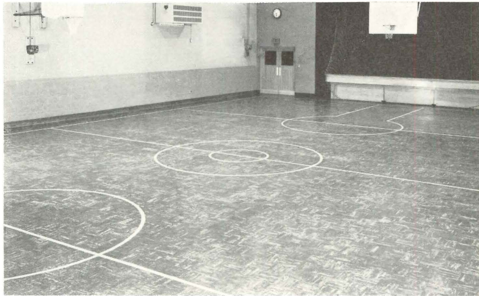
Gymnasium: "Flexachrome"/vinyl-asbestos tile/ inlaid game lines/ The Gunnery School, Washington, Conn./ Architects Sherwood, Mills & Smith/ The Tile-Tex Division, The Flintkote Company , 1232 McKinley St., Chicago Heights, Ill.
