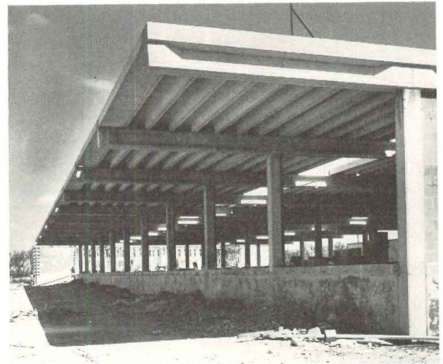
Figure 3—freight terminal utilizes long-span, channel-slab type of precast-roof construction. Channels rest on prestressed girders.
