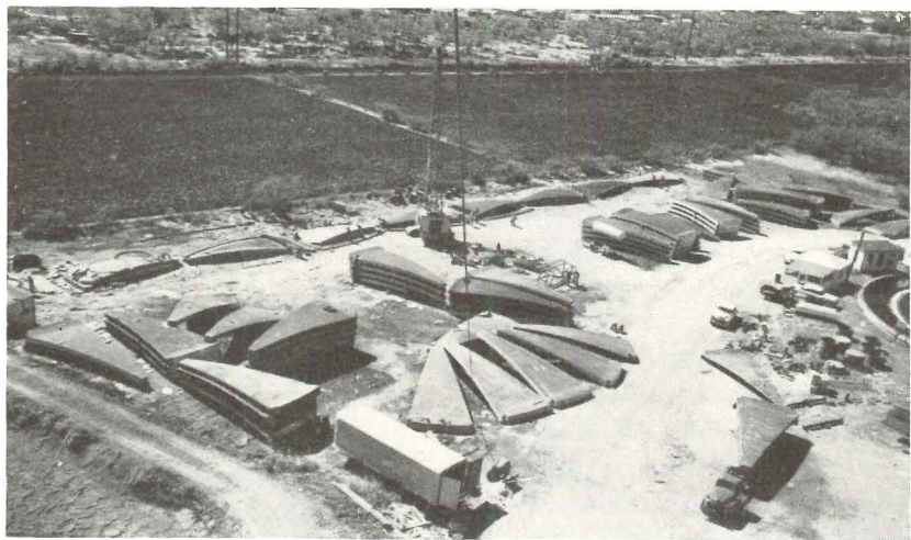
Figure 17—erection of thin-shell segments. A top compression ring was cast later (bottom)
