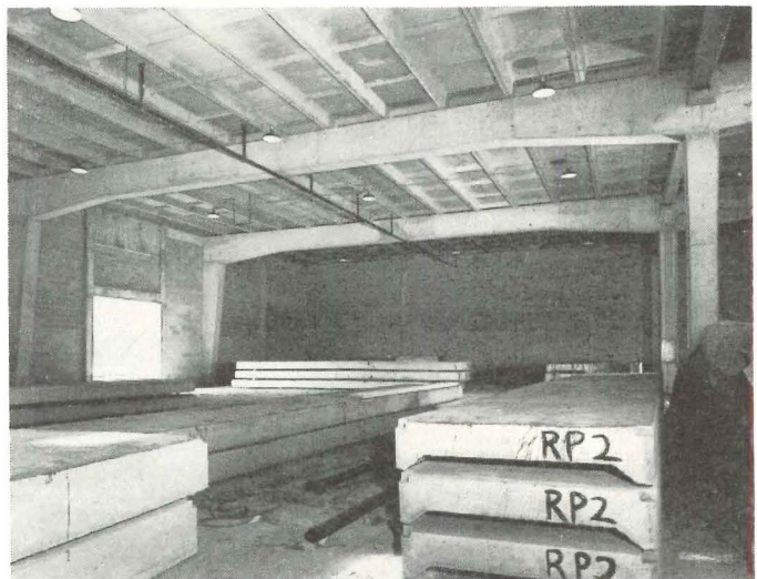
Figure 6—channel slabs shown in photo (above) were cast at job site (left).
