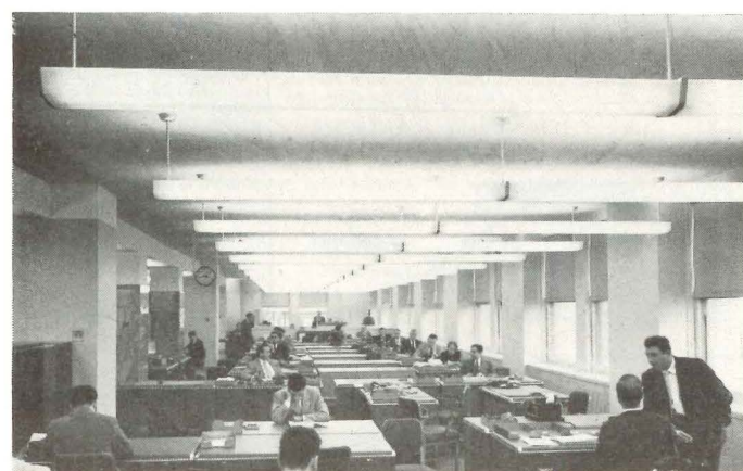
Figure 5—metal enclosures extending between columns conceal perimeter air-conditioning units (below).
