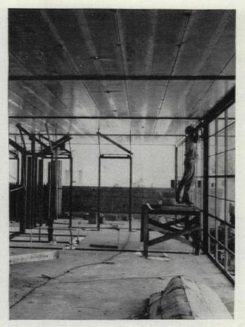
This construction photo of O'Neal School shows how Architect Drew uses the fast erection of Fenestra Building Panels and curtain walls of Fenestra Galvanized-Bonderized Steel Windows to close in a school quickly. This allows other trades to work "indoors". Contractors on Drew jobs can eliminate "down time" for weather as a contingency.
