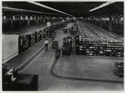
Order-filling area for immense wholesale drug warehouse serving 3000 customers with almost 35,000 items. "Towveyor" line pulls carts from one section to next. Shelving unit (left) demonstrates rear-feed principle which assures complete rotation of stock. Aisle for picking is open and order fillers are not impeded by stock replenishment men or loose cartons. Robert Montgomery Brown, Architect.
