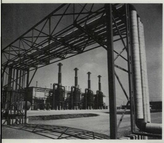
The joining of butadeine, styrene, and other essential chemicals to produce synthetic rubber is a manufacturing process involving precise control of temperature and pressure. The plant illustrated, south of Los Angeles, Calif., was built by the Ford J. Twaits Co., Construction Engineers; J. Gordon Turnbull, Inc., Consulting Engineers. New structural forms inevitably result from functional housing of such specialized processes.
