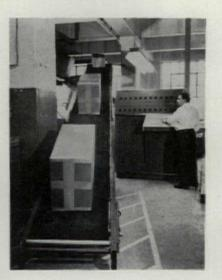
Waiting time for orders is greatly reduced at this lunch counter (right). Each waitress (one per bay) has tel-autograph device that transmits customer's order to kitchen. When order is prepared, it is brought by belt conveyor to waitress' station; signaling device automatically announces that order is ready for customer. Office of James E. Edmunds, Jr. and Ketchum, Giná & Sharp, Associated Architects.
