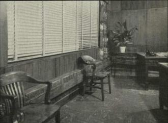
DUNHAM THERMO VECTOR RADIATION, painted to simulate wood paneling in modern office building, runs full length along outside walls, minimizes wall streakage.
