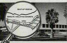
ZONOLITE Concrete over metal deck. Picture of Phoenix Public Library, Phoenix, Ariz. 21/2 inches of Zonolite Stabilized Concrete Aggregate; 1:6 mix. An insulating, fireproof, rotproof deck. Arch.: Alden B. Dow
