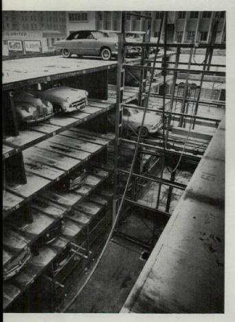
Automatic Parking Garage, (above and top right) Los Angeles, Calif. Kenneth N. Lind, Architect. Average parking time at this garage has been reduced to 38 seconds per car, thanks to a parking elevator which operates as a traveling joist. A projecting dolly moves cars in and out of their parking stalls. Cars can be locked by owners since all operations are done mechanically by elevator. Structure is of reinforced concrete and masonry.
