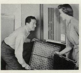
Fiberglas Dust-Stop\* Air Filters are key factors in assuring comfort and cleanliness in forced air conditioners. Dust-Stops are extra efficient because they trap dust, dirt and pollen all through the filter . . . not just on the surface.
