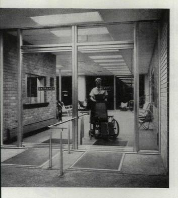
HERCULITE DOORS, equipped with mat-operated Pittcomatic hinges
