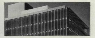
Fixed vertical louvers of Alcoa Aluminum on east-west elevations, horizontal on north-south. Cantilevered three feet away from building to block sunrays.
