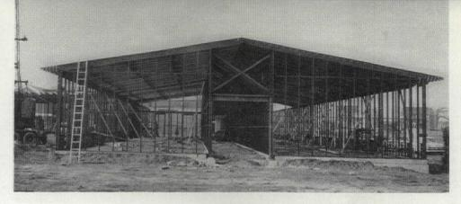
Using Penmetal light-steel structural sections, this school (above) was erected at a cost of \$13.65. Steel members for loadbearing partitions and roof joists were shop-fabricated into panels-some 32-ft longand trucked to job site. Penn Metal Co., Inc., 205 E. 42 St., New York, N. Y.
