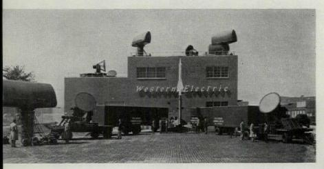
NIKE, anti-aircraft guided missile, requires highest degree of electronic control. Radar mechanisms (left) track weapon's flight, permitting technicians at control panels (below) to maintain contact with missile. When almost in vertical position, booster charge starts NIKE on its supersonic quest for a flying target. After initial thrust, lower portion is expended and missile proper continues toward target guided by its electronic brain.
