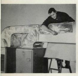
Fiberglas Duct Insulation (1) prevents excessive the gain in ducts; (2) silences the sound of air movement; (3) prevents condensation on cool ducts. Fiberglas makes a complete line of duct insulations—rigid or flex-ble, faced, sprayed, or uncoated.
