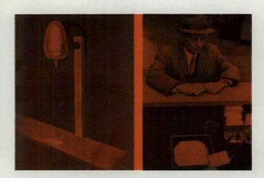
Closed-circuit TV speeds banking operations (left). On request from a branch bank, a balance, customer's signature, or whatever record may be wanted is placed under a football-shaped camera (General Precision Laboratory, Inc.) at the bank's headquarters-blocks or even miles away. The picture appears on the branch-bank teller's individual TV monitor, for verification. Duplicate records are thus avoided, and tellers are never required to leave their stations.
