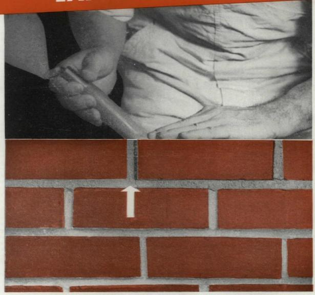
GOOD workmanship is one of the most important factors in preventing leaky brick walls.
