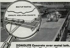
Photo of Luthe Hardware Company, Des Moines, Iowa. Fireproof deck was poured in place, cutting days off production schedule.
