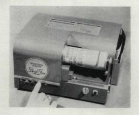
A miniature, facsimile-telegraph machine, called Desk-Fax (right), is used by telegraph customers to send and receive telegrams in picture form. Approximately 26,000 of these machines are presently in use and serve to connect customers offices directly with machines in central telegraph offices (below). Like Desk-Fax, machines at the "facsimile center" are capable of sending and receiving messages.
