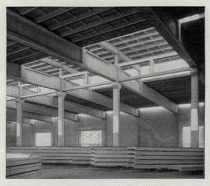
Roof constructed of precast concrete channel slabs resting on prestressed girders and precast monitor frames. Warehouse designed by the office of the late J. H. Davies, consulting structural engineer. Structural engineer was James R. Bole of Long Beach, Calif. Contractor was Johnson-Western Constructors of San Pedro, Calif.
