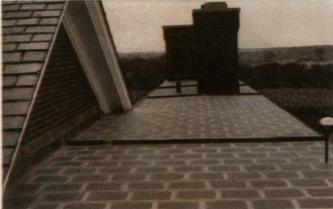
16" x 18" Copper "pans" of easily soldered copper were permanently applied on the horizontal section of the roof. Note expansion joints.
