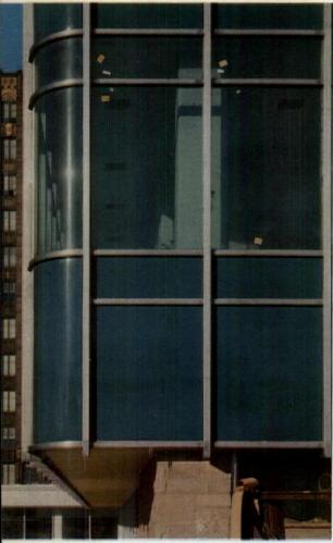
The interlocked steel curtain wall panels are assembled to the building with steel anchors, bolted at top and bottom of the spandrel beam.
