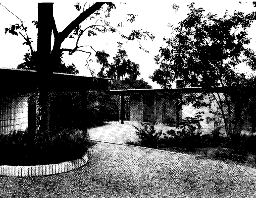
The structural system is composed of steel T columns, 16 ft o.c., supporting 30-ft steel WF beams. Wood joists (2"x12"), 16 in. o.c., frame between beams; with 2"x2" furring strips on top for through ventilation. L. F. Martin-BUILDER, Inc., was General Contractor. Photos: Alexandre Georges
