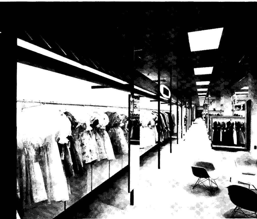
Perimeter wall fixture (above) employs 6½"-wide boards, spaced 1" apart, to emphasize the individuality of this department. Mirrors are directly mounted on metal uprights.
