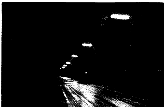
Figure 8—medium-traffic street (private industrial roadway) in East Cleveland, Ohio, with four fluorescent lamps (21,000 total lumens) per luminaire; 25-ft mounting height, 100-ft spacing, 1.0 ft-c average maintained. Wet street shows large area patterns of reflected brightness on pavement.
