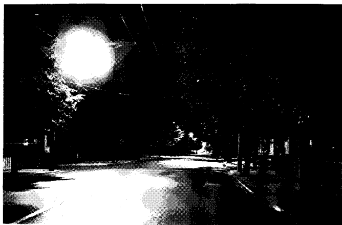
Figure 6—medium-traffic street in Malden, Mass., with mercury lamps; 15,000 lumens, 28-ft mounting height, 110-ft spacing. Luminaires located to reduce shadows from heavy tree foliage.
