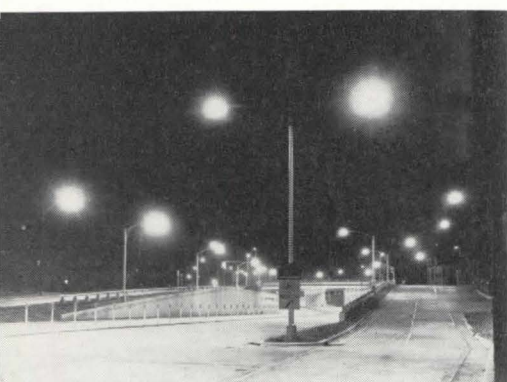
Figure 10—arterial street in San Jose, Calif., with filament lamps; 10,000 lumens, 28-ft mounting height, 140-ft spacing between pairs of opposite units.
