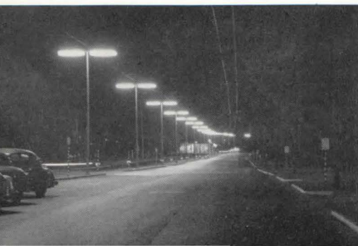
Figure 11—arterial divided roadway just beyond shopping center in Oakwood, Ohio, with four fluorescent lamps (21,000 total lumens) per luminaire; 30-ft mounting height, twin-mounted at 95-ft spacing. Average initial illumination 1.7 ft-c.
