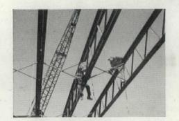
MORE SAVINGS IN LIGHTER FRAMING AND FOOTINGS are possible with the new Truscon Clerespan® Steel Joist. To meet all types of loading conditions, it utilizes a Warrentype truss. Joist depth is standardized at 18" to 48". Open webs provide passage for and concealment of ducts, pipes, electrical conduit. Send for new Truscon catalog, E-280, which gives you all the facts on Clerespan Steel Joists up to 96 feet in length.
