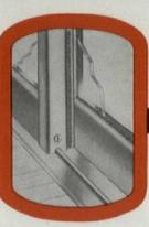
...Double Mohair pile weatherstripping at interlocking stiles, preventing air or water infiltration.
