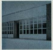
Sliding Doors of aluminum tubes and aluminum sheets roll sideways into compact pockets to allow maximum unrestricted indoor-outdoor space use.
