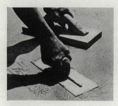
Latex concrete topping (above) which bonds to any clean, stable surface (even to one as smooth as glass) can be used for patching cracks in any concrete or masonry surface, for repairing stone or slate, for repairing brick or mortar joints, and smoothing asphalt-mastic surfaces. Can be applied as thin as 1/16" or as thick as needed. The Camp Co., 6958 S. State St., Chicago 21, 111.
