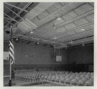
Bethlehem Longspan Joists span the gymnasium, giving uninterrupted, column-free space below.
