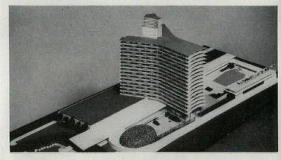
rear guest rooms. Utility tower at "Y" intersection will enclose elevators and stairs. Building will be fully air conditioned and heated. Architects are: Igor B. Polevitzsky and Johnson & Associates, Miami, Fla., and Manuel Carrera, Cuba.
