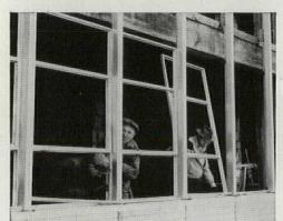
Here experienced Lupton crew men insert wall units between vertical mullions from *inside* the building, without scaffolding or special hoisting equipment. (They are designed to be installed from either inside or out.) Single Lupton contract provides single responsibility for manufacture and installation of curtain wall system.
