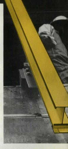
**Above:** The first I-shaped mullions of architectural bronze are set in place on the 53rd Street side of the East Wing. These are the longest extrusions— 26' 4"—used on the building.
