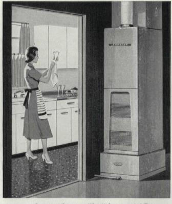
Are your homes without basements? This combination of a Carrier downflow type Winter Weathermaker with a Summer Weathermaker underneath is perfect if you put your ducts in the slab or crawl space. Takes very little space in the house. Gas or oil fired.
