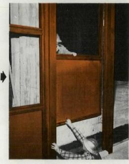
SHOWING ONE OF THE 4,554 PANELS each containing a spandrel sheet of Revere Architectural Bronze, weighing a total of 325,000 lbs.
