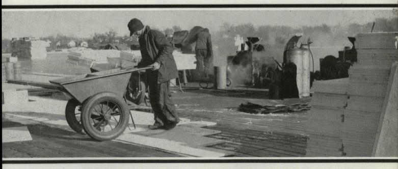
**Better, faster methods** make present-day roofs a better "buy" than ever before. But the picture above shows the need for an insulation material that can safely withstand heavy loading. Heavy LP gas cylinders, asphalt kettles, big
