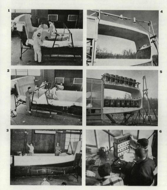
Molded modules are cantilevered in pairs from a 16-ft square central utility core to form four 16-ft square rooms. Completion of the full-scale house is scheduled for June in the Tomorrowland area of Disneyland at Anaheim, Calif.
