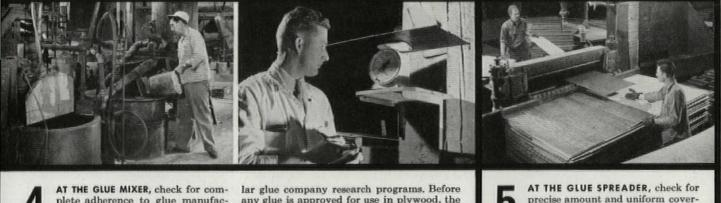
AT THE GLUE MIXER, check for complete adherence to glue manufacturer's mixing directions. Special formulae developed by million dollar glue company research programs, Before any glue is approved for use in plywood, the manufacturer *must* submit products for performance testing under factory conditions. AT THE GLUE SPREADER, check for precise amount and uniform coverage of adhesive. Check proper curing time, recheck veneer condition.
