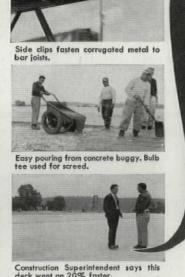
This type of joist used where span exceeded 25 ft.
