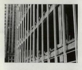
Vertical mullions of extruded aluminum that act as the "organizing element" of the wall are bolted to the galvanized clips. Slots in the angle clips and galvanized clips allow extremely accurate positioning of the mullions, regardless of structural irregularities.
