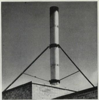
The Van-Packer is a cylindrical stack of 3-foot long centrifugallycast refractory sections, cemented one on top of another and secured with draw-up joint bands. Sections are of vermiculite-concrete with aluminum outer jacket.
