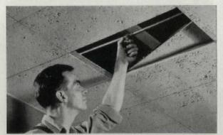
**Reach through** to work-and when the tile is replaced, it becomes part of the unbroken ceiling again.
