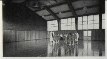
The concrete, three-hinged arches of the multi-usegym (above) become the pattern of the finished design; flooring is maple.
