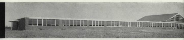
Fowlerville High School, Fowlerville, Michigan, is designed with interior load-bearing masonry walls and Fenestra Acoustical-Structural "D" Panels to reduce structural steel requirements to a minimum. Total costs for this 41,000 square foot school were approximately \$11.00 per square foot . . . an economical figure for high school construction in this area.
