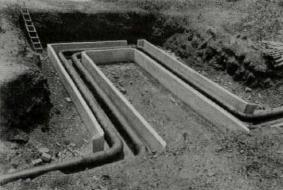
Figure 7—expansion bends in supply and return lines for a HTHW system. American Hydrotherm Corp.
