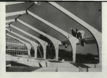
All support elements (above) are provided by single, self-sufficient wood units, made of glued-laminated Southern Pine. Each structural section is fabricated in two parts—two units forming arch to carry roof and wall loads; third unit is beam, to carry floor load, fitted in brackets about 2' above base of arch. When bolted, units form single section. Southern Pine Assn., P.O. Box 1170, New Orleans 4, La.
