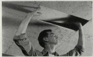
Simply lift up the acoustical tile at the access point to get at utilities and ductwork.
