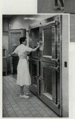
**FOUR-WINDOW** refrigerator front—also stainless steel clad—glazed with three thicknesses of plate glass  $\frac{1}{4}$ " thick. Sturdy hardware is chromium plated heavy cast bronze.
