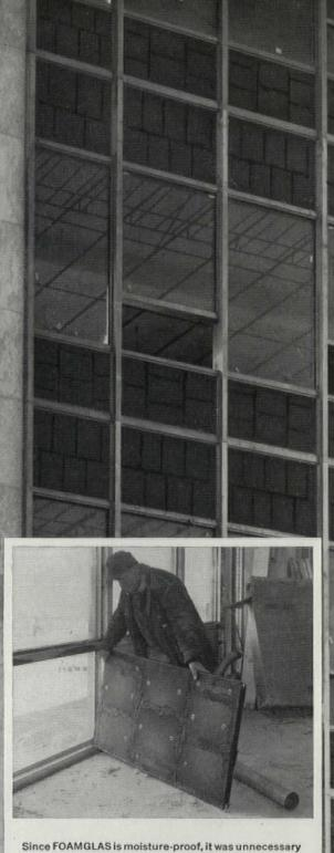
to protect it from the weather during installation . . . as shown by this exterior view taken during construction of the new American Hardware Mutual building. Inset shows spandrel backup pan containing FOAM-GLAS about to be installed in curtain wall mullions.
