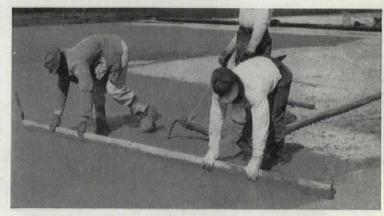
EFFECTIVE INSULATION. Inert insulating concrete is one of the most permanent, desirable types of roof insulation. Rigidity of Tufcor system provides a firm base for built-up roof. Low dead load of finished Tufcor system is 4 to 6 psf less than most types of roof construction, requires less structural steel. Permanence, low maintenance of system plus low insurance premiums assure savings to owners.
