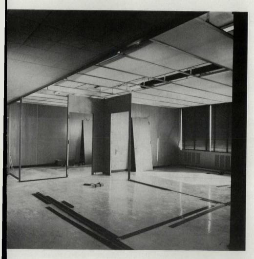
A panel, rather than post-and-panel, system constitutes the movable office partitioning. Components include 1¾"-thick panels with Korina wood veneer and fire-proof core; plain panels framed in aluminum extrusions; corridor panels of polished plate glass. Ceilings are luminous vinyl plastic in office spaces and perforated-metal pans in corridors; flooring is light beige, marbleized rubber tile.
