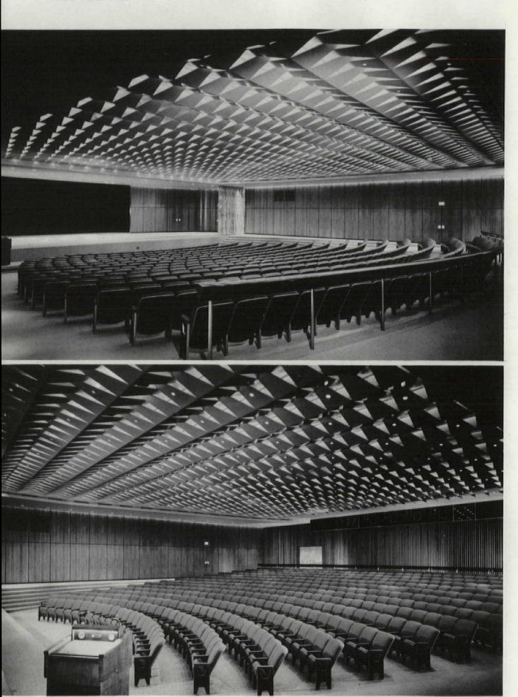
Teak surfaces the walls of the 500-seat management conference room (acrosspage), whose stage is equipped with a turntable. The ceiling is composed of bent, diamond-shaped panels of steel that conceal both incandescent and fluorescent lamps, which allow a wide variety of light quality and intensity. The floor cover is dark-gray carpeting.
