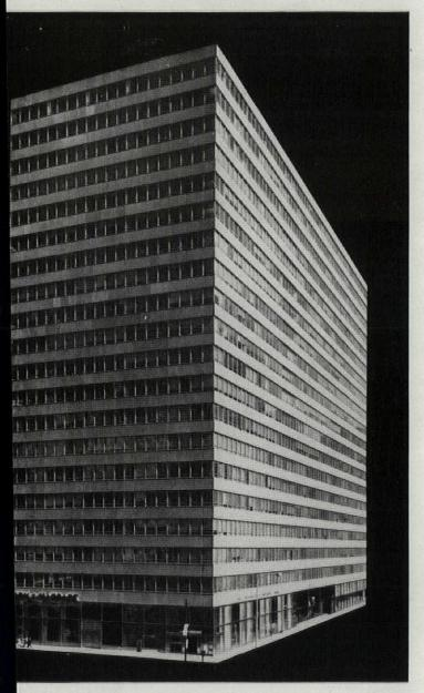
3 PENN CENTER, Philadelphia, Pa. Architects: Emery Roth & Sons. Contractors: Caldwell-Wingate Construction Co. Combination fixed and ventilator windows adapted from a standard Lupton design.
