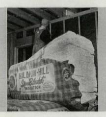
B-H Big Six batts are packed under compression to save builders' storage space — but see how they expand to the full six-inch thickness when the package is opened. This resilience is permanent! It is "builtin" by Baldwin-Hill's process of spinning molten minerals into long, fine, interlocking fibers that never settle into a compact mass.
