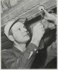
Automatic home fire-alarm system-providing simple, low-cost safety feature-operates on a small transformer easily installed in standard three-gang outlet box in bedroom (far left). Control panel, measuring 4\%" x 61/2" for surface or flush mounting-contains transformer, test button, and ringing bell. Automatic fire detectors are installed in typical attic and basement areas (left) and connected to control unit by ordinary bell wire. Edwards Company, Inc., Norwalk, Conn
