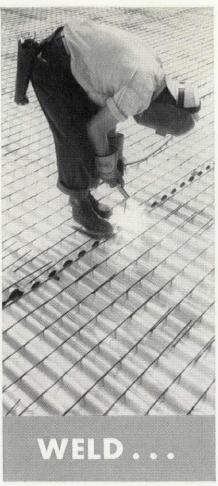
Welded in place, Cofar provides a safe, solid work platform for trades. Concrete crews move in days sooner. Cofar welding gives designers flexibility to meet local codes for lateral forces.
