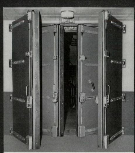
Jet engine test cell — inner and outer sets of double Jamison Sound Reduction Doors minimize extremely high sound levels.
