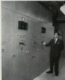
INCOMING SERVICE AT 13.2 KV is reably handled by easy-to-maintain Gmetal-clad vertical lift switchgear.
