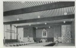
Rilco laminated wood beam sizes  $77' \times 11'' \times 34\%''$  and  $67' 4'' \times 7'' \times 34\%''$ .
