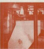
Wheeling SofTite Cop-R-Loy Galvanized Sheets were used for the 1,600 horizontal air distribution sections plus 62 vertical shafts.
