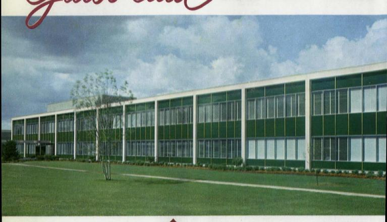
THE COMPLETE Pittsburgh system of curtain-wall construction is shown in this new building housing the National Carbon Company's Research Laboratory at Parma, Ohio. This system effectively utilized Spandrelte and Pittco 82-X with Pittsburgh's Solex® Heat-Absorbing, Glare-Reducing Plate Glass. Architects: Skidmore, Owings & Merrill, New York City; Contractor: Gilmore-Olsen Company, Cleveland.
