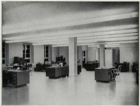
Here's an interior view showing a small part of the installation of Gold Seal Inlaid Linoleum. Actually, about 3½ acres of floor space are covered with this ½" burlap-backed "Veltone."
