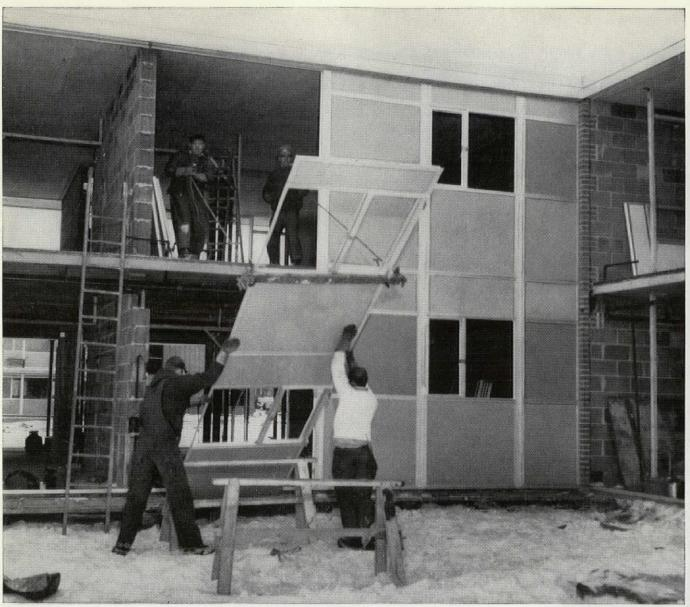
Workmen installing window walls made with Hasko-Struct<sup>†</sup> plastic laminated sandwich panels. Architect is Manson & Carver Associates, General Contractor is Christman Company.
