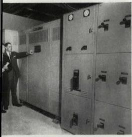
FLEXIBLE double-ended load center unit substation with integrated units furnishes highly dependable power close to load.
