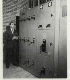
COMPACT low voltage switchgear and distribution switchboard protect low voltage side of "packaged power" system.
