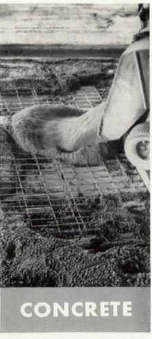
In monolithic slabs, Cofar offers composite action to resist concentrated loads and horizontal forces. For steel or concrete framing. Cofar underside may be painted for finished ceiling.
