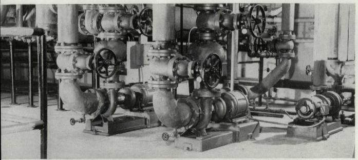
Battery of silent B&G Universal Pumps circulating a two-pipe, reverse return hot water heating system.
