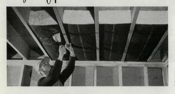
B-H Big Six batts in-stalled in lower-floor ceilings to eliminate the "tramp, tramp" and other noise from the up-stairs tenants.
