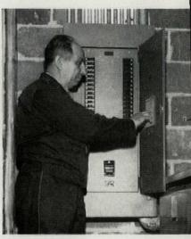
**SAFER** G-E panelboards with molded-cas circuit breakers are designed to occup little space, permit easy wiring. They are installed in wiring closets.
