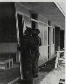
Prefabricated window wall sections are delivered to the job and stored in the building shells ready for quick, easy installation.
