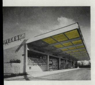
ve Thru Markets get double-duty, too, with Corrulux opies to protect their "stay-in-the-car" customers while smitting flattering light to all food display racks.... igned by W. G. Horn, Mecca Engineering Company.
