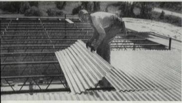
EASY TO PLACE. Tufcor sheets arrive at the job site bundled and cut to fit framing. No measuring or cutting is needed! After sheets are plug-welded in place, they provide a strong structural deck and a convenient work platform for trades. In the finished roof system, Tufcor acts as a vapor barrier, keeps insulating concrete dry so it maintains its insulating properties, saves on costly fuel bills.
