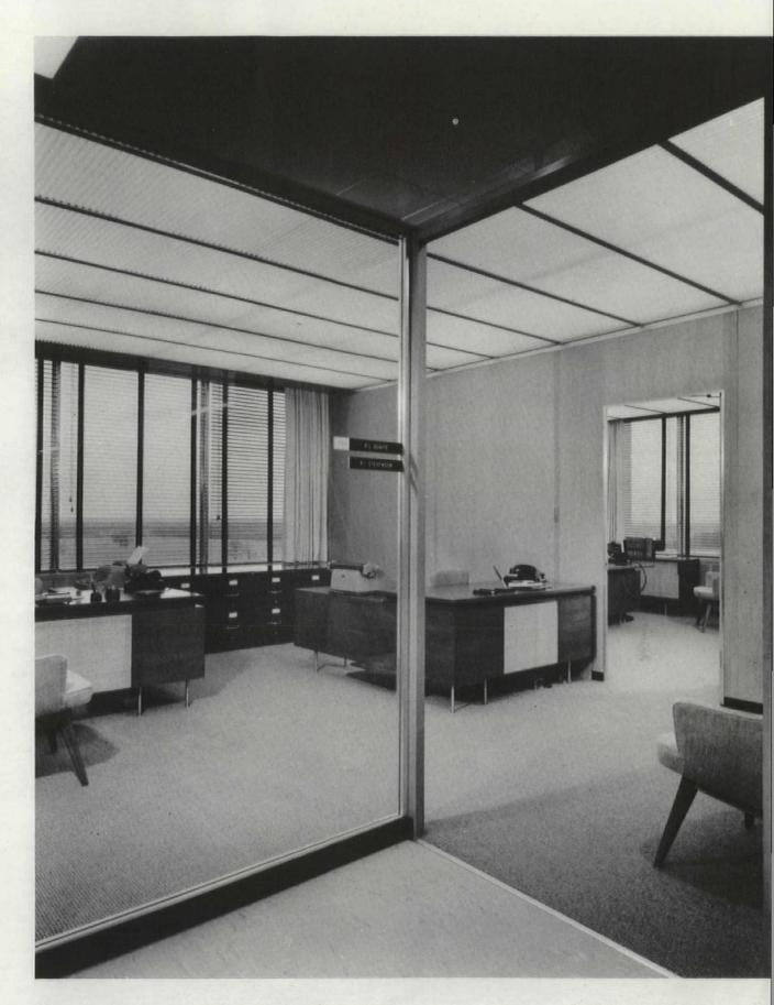
Offices and office suites are very largely on display, due to the use of plate-glass panels as the standard corridor-wall unit. The modular partition elements are clearly shown in the pictures on these two pages—fireproof Korina veneer units where a solid wall is wanted, and aluminum-framed panels in both clear and textured glass. For the more elaborate office suites, carpeting, rather than rubber tile, is used for the floor surface.
