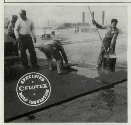
Permanently efficient insulation . . . plus important on-the-job advantages: Rugged, hard-to-damage. Lightweight, easy to handle and apply. Cleancut, snug-fitting edges insure flush contact at joints. A smooth, solid base for roofing felts. Ideal mopping surface, excellent bond. Exclusive Ferox® treatment protects effectively against dry rot.
