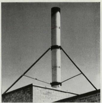
The Van-Packer is a cylindrical stack of 3-foot long centrifugallycast refractory sections, cemented one on top of another and secured with draw-up joint bands. Sections are constructed of refractory material with aluminum outer jacket.
