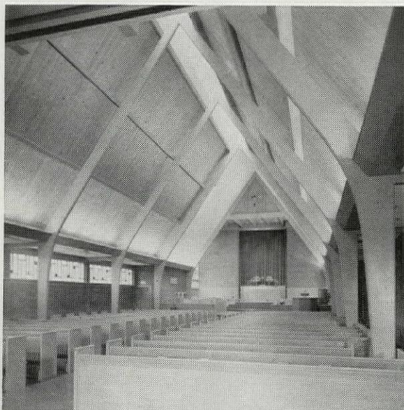
Addition to All Saints Episcopal Church, Portland, Oregon. Architect: Stuart B. Mackford, Oregon City, Oregon. Contractor: Anfelt B. Hanson Company, Portland, Oregon. Arch span: 34'; center height 33'4"; 3 arches 5 1/4" x 7" x 17" at tangent point; 2 arches 5 1/4" x 7" x 10" at peak base.
