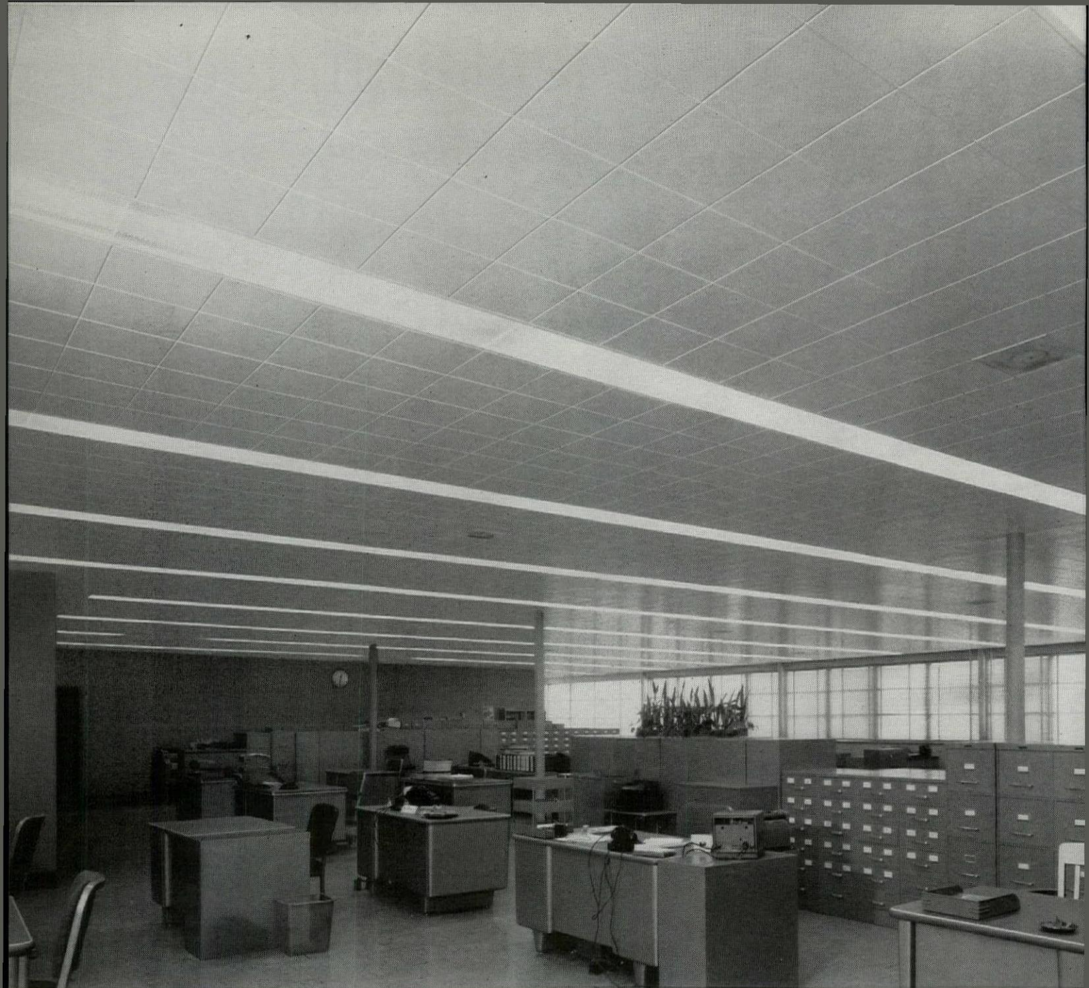
Recessed type lighting complements the appearance of this suspended acoustical ceiling of Armstrong Arrestone. VANDERCOOK & SONS, INC., CHICAGO, ILLINOIS. JOHNSON & JOHNSON, ENGINEERS-ARCHITECTS, INC. AIRTITE, INC. ACOUSTICAL CONTRACTOR.
