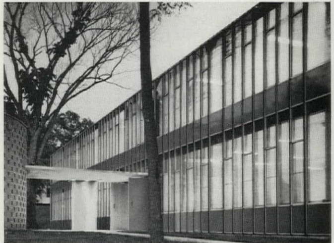
COLLEGE OF THE BIBLE , Drake University, Des Moines, Iowa. Architects: Eero Saarinen & Associates, Bloomfield Hills, Mich. Contractor: Fane F. Vawter Co., Des Moines, Iowa. LUPTON curtain-wall units—one-third the thickness of masonry—go up fast, leave extra square footage indoors.
