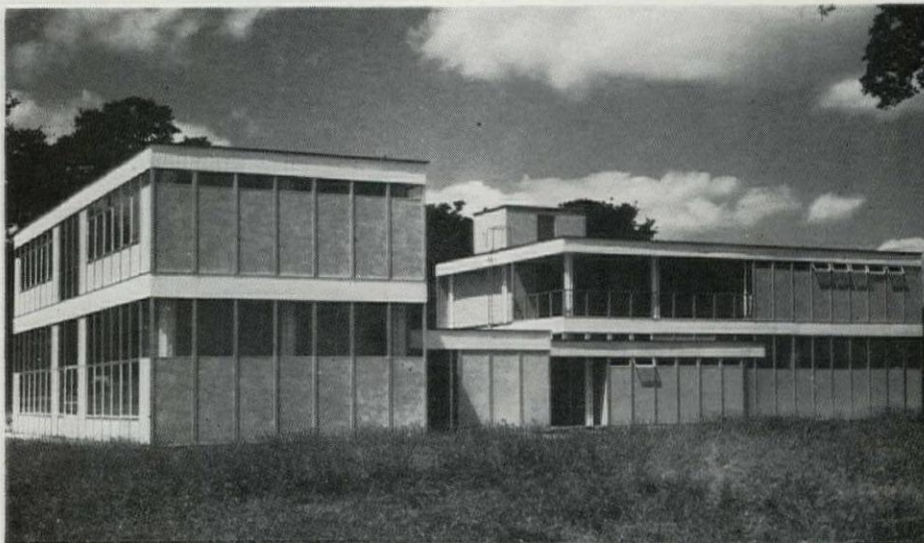
Figure 3—Clarendon secondary school, 1950 prototype has 3'-4" module. Exterior view shows repetition of aluminum mullions at modular intersections; wall panels are cellular plastic. Construction photo (acrosspage) reveals cruciform steel columns and open-web joists. Hertfordshire County Architect.
