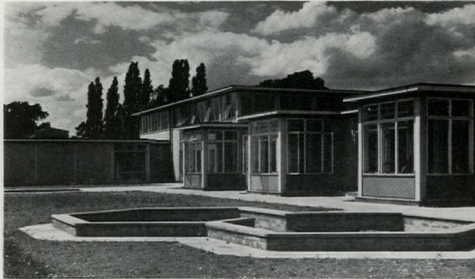
Figure 2—Morgan's Road primary school, a unit of the 1948-49 program. View of infants' wing shows vertical cladding blocks that permit window openings which are not full-bay width. Plan (acrosspage) indicates flexibility of perimeter that is possible and economic within limits of a 8'-3" module. Hertfordshire County Architect.
