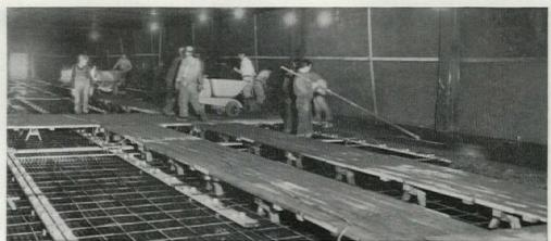
Placing concrete floor made with LEHIGH EARLY STRENGTH CEMENT. Quick-curing concrete permitted early use of this floor for storage of construction materials.
