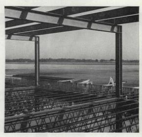
CONSTRUCTION of Cleveland Air Terminal's West Concourse, shown above, was speeded by use of Truscon "O-T" Open Truss Steel Joists. These lightweight, strong, fire-resistant floor and roof supports lessen time and labor costs. They save material in supporting framework and foundations. See Sweet's File for specifications on "O-T" Steel Joists and other quality Truscon Building Products. Or send us the coupon.
