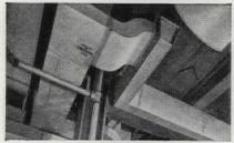
Ducts made of SOFTITE Cop-R-Loy form quickly without preliminary cutting.
