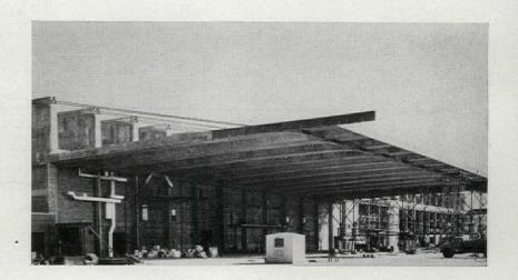
Construction-progress photo (above) shows soffit of corrugated-concrete-slab roof after metal forming has been removed. Section through slab (below) indicates slope and dimensions of end and typical slabs.
