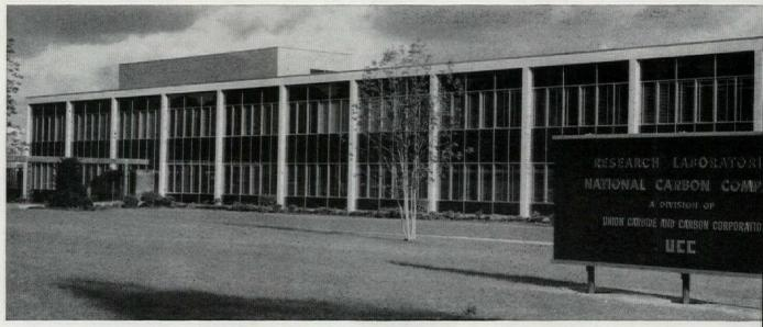
The graceful, modern appearance of this new structure is immediately apparent in this exterior view of the front. Here, the full effect of the Solex and Spandrelite curtain wall is completely realized.
