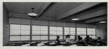
GOOD ACOUSTICS. Tests conducted by Riverbank Acoustical Laboratories indicate that Structur-Acoustic system with  $2\frac{1}{2}$ " slab provides Noise Reduction Coefficient of .80. Clean, corrugated underside of Structur-Acoustic reflects light, can be painted to matching color scheme. Hard surface won't dent, stays attractive. Heat loss is kept to minimum with U factor in excess of 0.14. Firesafe system protects both building and contents, helps reduce owner insurance costs.
