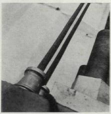
Detail of pylons (above left) shows pilaster, bulb, and strands. Pilaster was designed to stabilize edges of walls as well as to carry load to ground. Emulsion-type acrylic paint was sprayed on top surfaces of roof slabs.
