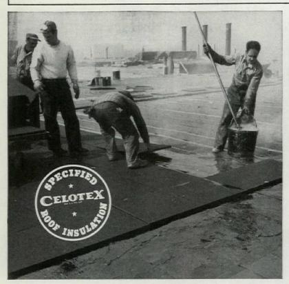
Permanently efficient insulation . . . plus important on-the-job advantages: Rugged, hard-to-damage. Lightweight, easy to handle and apply. Cleancut, snug-fitting edges insure flush contact at joints. A smooth, solid base for roofing felts. Ideal mopping surface, excellent bond. Exclusive Ferox® treatment protects effectively against dry rot.
