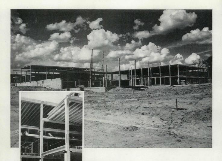
Allison-Erwin Warehouse and Office built with deflected strand precast prestressed concrete members fabricated and erected by Concrete Materials Incorporated, Charlotte, North Carolina. The seven-wire uncoated stress-relieved prestressed concrete strands were manufactured by Roebling.
