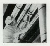
The makers of Hellmann's Mayonnaise first used Styrofoam\* (a Dow plastic foam) in 1952. That was to insulate egg-storage rooms. The results have been so satisfactory that when Best Foods planned a new unit for making salad oil, Styrofoam was specified for 40° insulation in the winterizing cells (see illustration).
