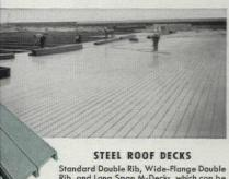
Standard Double Rib, Wide-Flange Double Rib, and Long Span M-Decks, which can be furnished with perforated surface and fitted to provide an efficient acoustical ceiling.
