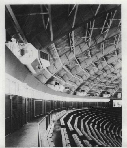
Diameter of the hard maple playing floor is 132 ft-large enough for an exhibition tennis court, including backstops, or two basketball courts. Topping the 38-ft dome structure (that houses ventilating fans and floodlights) at the peak of the big dome is an 8-ft-diameter plastic skylight.
