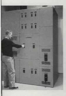
Typical switchboard: positive breaker handle identification shows when circuit has been interrupted.
