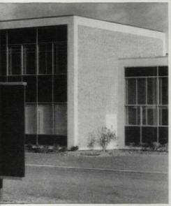
This view shows the SOLEX wall area in the cafeteria. SOLEX keeps interiors more comfortable by reducing solar glare and heat entering a building.
