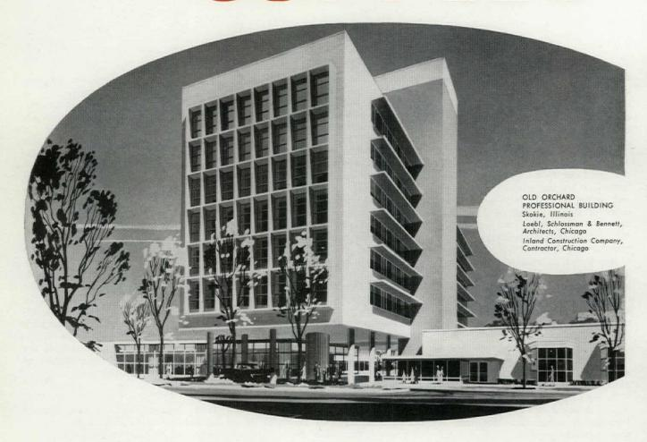
Here's another excellent example of how effectively aluminum curtain walls meet contemporary construction requirements.
