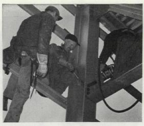
AIR TERMINALS and other structures often go up faster and at less cost with Republic High Strength Bolts, Installation can be made without waiting for specialized riveting crews. Bolted construction provides a more positive and reliable clamping force than is ordinarily possible with rivets. The greater strength of a bolt gives it higher fatigue-resistance. Mail coupon for more facts on Republic High Strength Bolts.
