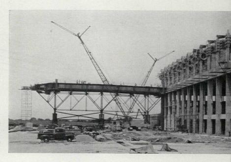
Before being anchored to ends of cantilevered slabs, strands are coiled at tops of pylons (right). Slabs are jacked and raised from the forms, before removal, to accommodate elongation of strands.
