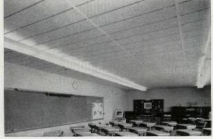
The clean, unbroken lines of the Panelcoustic ceiling...with only cool air to tell you the air conditioning is here, too!
