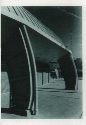
The elliptical, built-up, welded girders span 130 ft from hinged foundations to a circular girder at the crown, 10 ft in diameter. The ribs consists of a web plate and two flange plates, with bulb tees for stiffeners. Wood-chip concrete boarding is the sheathing, and the roof surface is 40-lb standing-seam metal.
