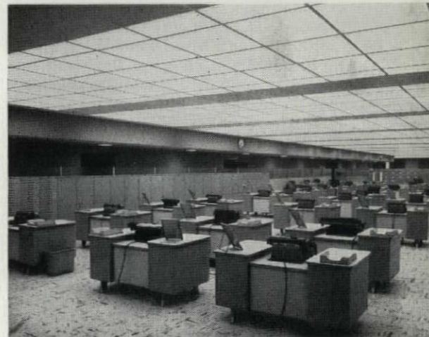
GLARE-FREE 277-V FLUORESCENTS in unique fixtures achieve ideal brightness ratio for office areas, create savings by combined lighting system, power source.
