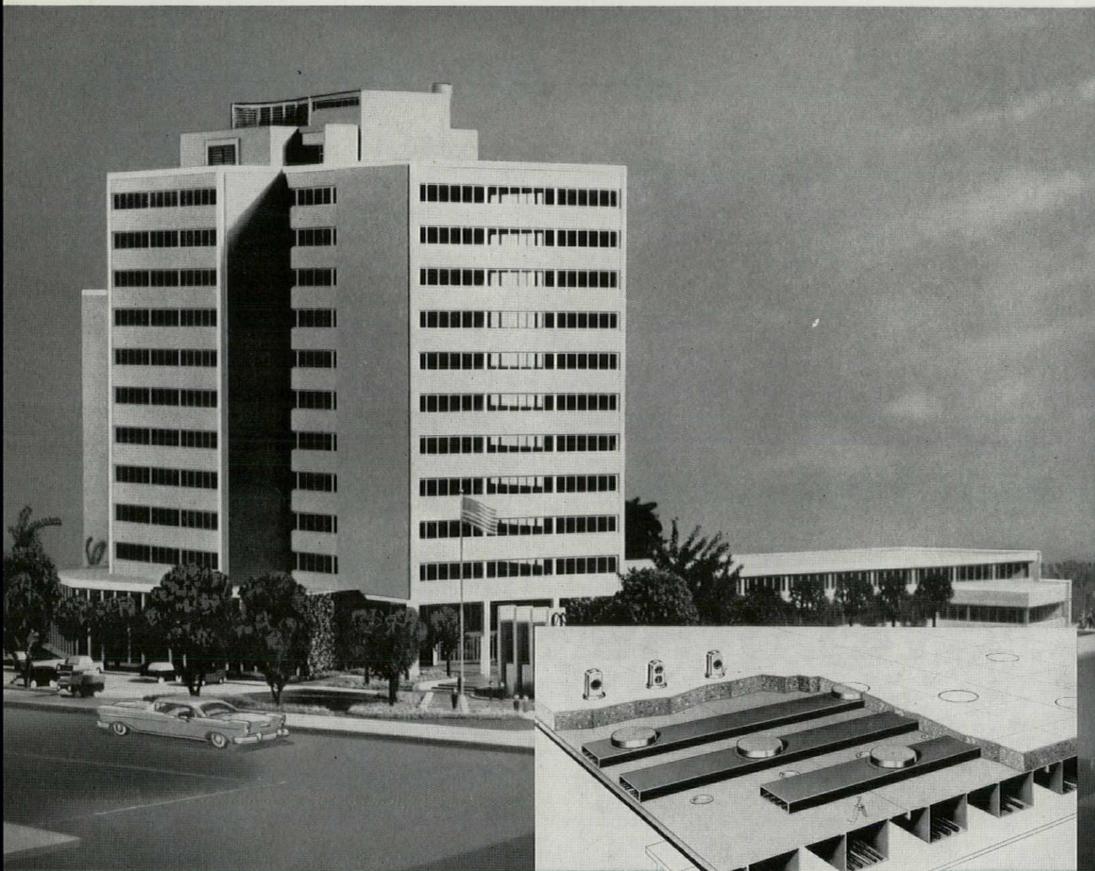
Sedgewick County Court House and Welfare Building, Wichita, Kansas. 196,000 Sq. Ft. of Mahon M-Floors and 15,000 Sq. Ft. of Mahon Steel Roof Deck will provide the Electrified Sub-Floors and the Roof of this modern building. Thoma-Harris-Calvin & Associates, Architects. Martin K. Eby, General Contractor.
