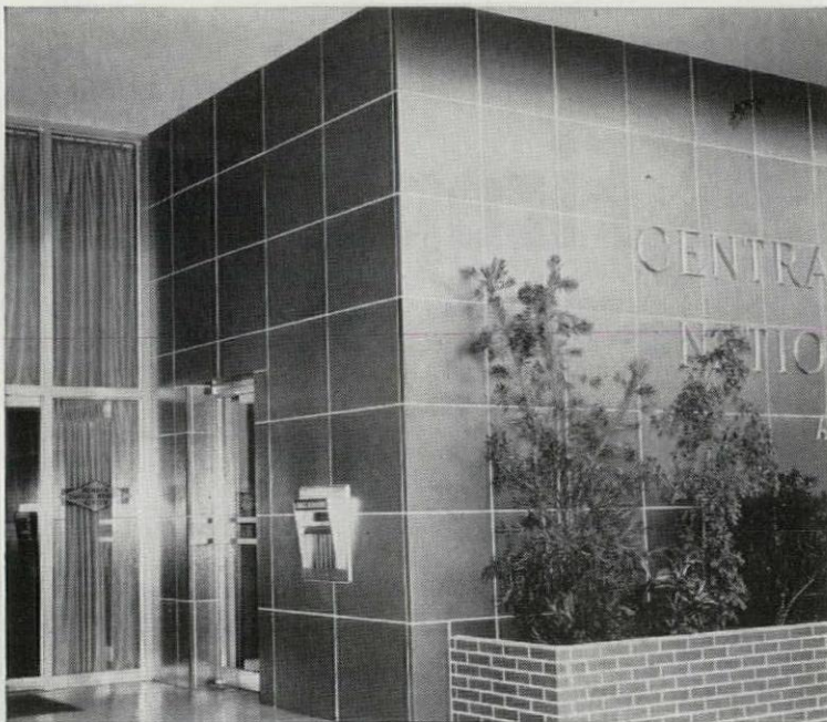
CENTRAL BREVARD NATIONAL BANK COCOA, FLORIDA Stevens and Sipple—Architects Ceramic Veneer units 24" x 24" x 2" were specified for exterior facing. Color is mottled emerald green.
