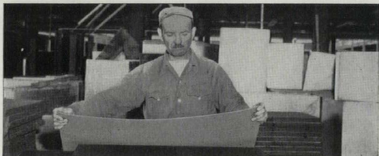
Flexible flashing is quickly adhered to FOAMGLAS blocks to form panel-size units of insulation. Two men easily handled all cutting and assembly operations for the insulated spandrel panels.
