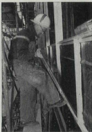
Application of Spandrelite completes the installation. Five men assembled and installed all of the spandrel panels.
