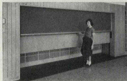
R-W No. 775 "VERTICAL-LIFT" Wardrobes . . . available in Aluminum or Wood Veneer in either a solid or hollow core design, electrically or manually controlled. A modern wardrobe combining maximum strength with dependable, easy operation.
