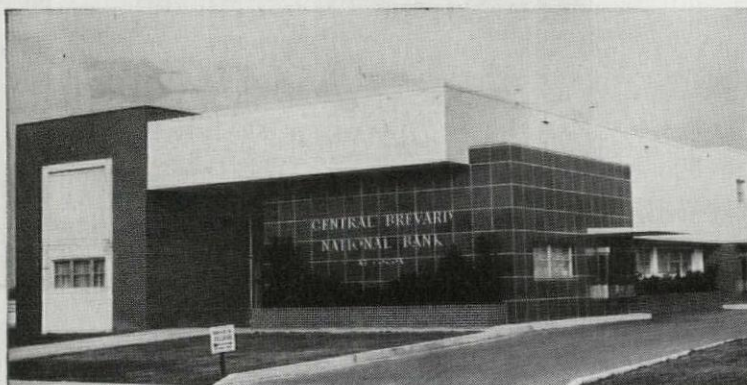
CENTRAL BREVARD NATIONAL BANK COCOA, FLORIDA Stevens and Sipple—Architects Ceramic Veneer units 24" x 24" x 2" were specified for exterior facing. Color is mottled emerald green.
