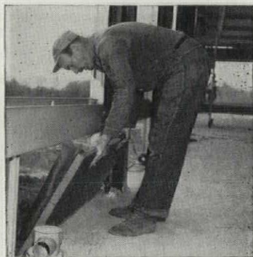
FOAMGLAS panel units are quickly and easily installed in spandrel areas before the facing is applied.
