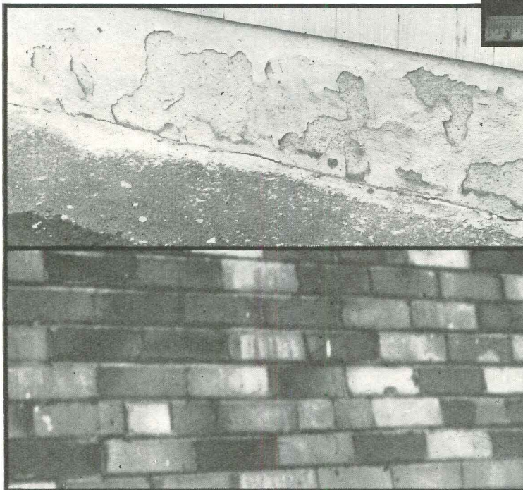
Efflorescence
