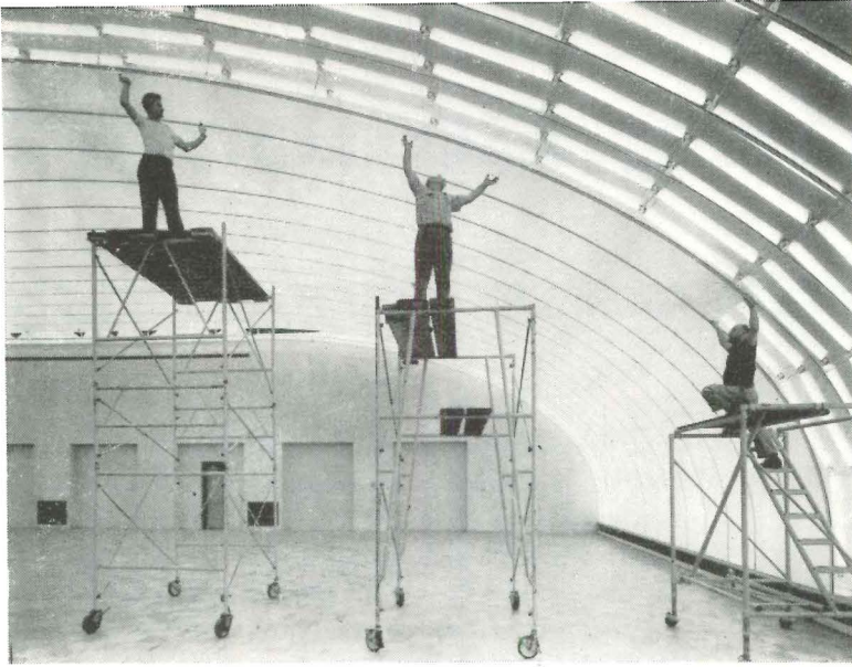
A luminous ceiling of Bakelite rigid-vinyl sheets (above) encloses Chrysler's styling showroom at Highland Park, Mich. Designed and manufactured by Wakefield, the ceiling follows a parabolic curve to the floor, eliminating shadows under mock-up cars and offering a simulated horizon to check automobile silhouettes. Maximum light averages 240 ft-c at working level. The Wakefield Co., Vermilion, Ohio.
