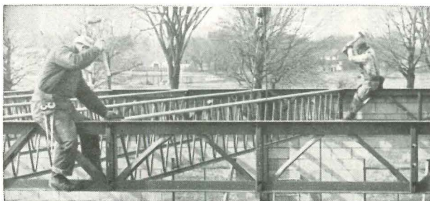
Steel Erection — V-LOK is an exclusive Macomber interlocking framing system that requires no on-the-job bolting, riveting or welding.
