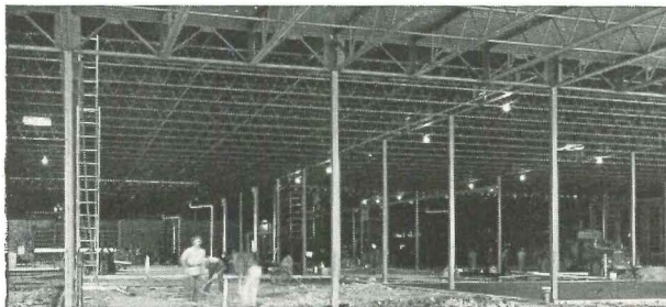
Under Roof — V-LOK steel framing provides the ideal support for Macomber steel deck roofing. Workers were able to proceed with interior construction without delay.
