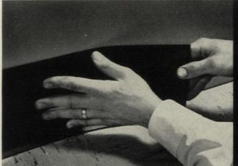
QUICK SETTING. 3M Cove Base Adhesive holds base firmly in place immediately after application without shoring. Bond can be completed up to 15 minutes after applying the adhesive. One gallon covers about 300 lineal feet of 4-inch material. Ideal for rubber, vinyl, asphalt.
