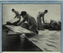
ROOFMATE better built-up roofs—Specially designed for built-up roofs, this new roof insulation board has high compressive strength, permanent insulating efficiency, long life. It can be easily installed, easily mop-coated with asphalt or other standard coating materials.
