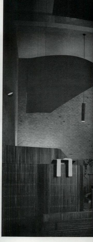
The center of worship is bordered by a slatted wood screen that, with its backing of sound-absorptive material, contributes to the excellent acoustics of the room.
