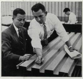
B-deck has wide ribs for maximum strength and rigidity. Safely carries normal loads over spans up to 10'. Wide purlin-spacings cut framing costs.
