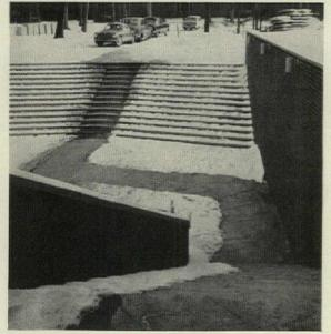
pipes. Described are lead-jacketed asbestos heating cable, designed to dissipate heat at rate of seven w per ft when used in proper lengths at correct voltages; lead-sheathed Flamenol jacketed cable, of rugged construction, designed specifically for snow melting, rated at 10 w per ft; siliconerubber cable, rated 10 w per ft in practically any installation.
