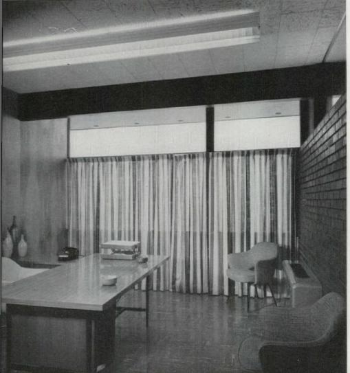
The building interiors have floors of terrazzo (corridors); rubber tile (offices); and ceramic tile (washrooms). The typical private office has one wall of brick; one of glass; the others of birch, walnut, or fir plywood. Ceilings throughout are of acoustical tile. Partitions have staggered studs with 2-in, blanket insulation. Interior spaces are lighted by plastic domes in the roof.
