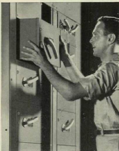
Individual switch units, even whole sections, can be added or changed as requirements dictate.
