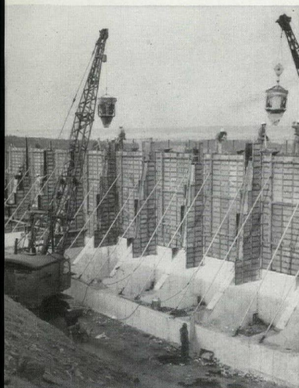
CONCRETE RETAINING WALLS reach 36 feet high over much of the 10,000 foot wall length. Tallest pours were made by giant overhead crane. Walls required approximately 24,000 cubic yards of Pozzolite concrete—a placeable mix of 2" to 4" slump with design strength of 3,000 psi. Contractor: T. F. Scholes, Inc., Reading, Pennsylvania. Concrete Contractor: Long Construction Co., Denver.
