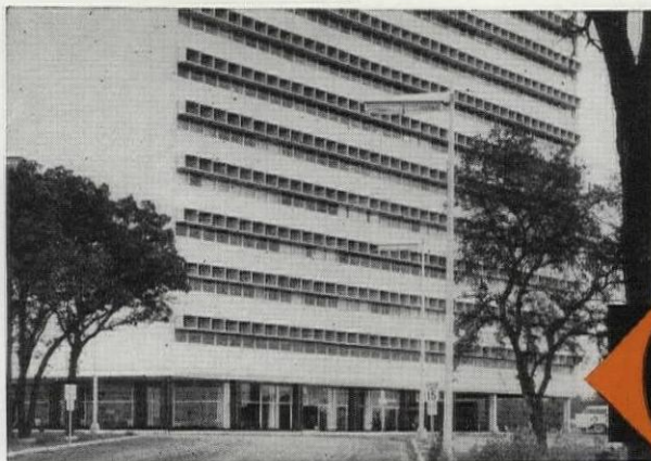
Exchange Bank and Office Building, Dallas, Tex., featuring all welded steel tube curtain wall framing. (Lane, Gamble & Assoc.)
