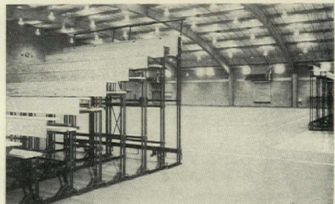
rigid flooring that would take abuse, consisting in general of 2" gravel sub-base; a 5" Bitumuls penetration Macadam base; and surfacing with 1 1/2" of Laykold mastic mix and Laykold colored surface.
