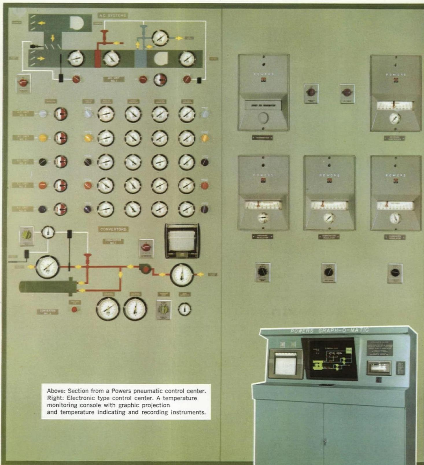
Above: Section from a Powers pneumatic control center. Right: Electronic type control center. A temperature monitoring console with graphic projection and temperature indicating and recording instruments.
