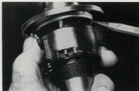
3 Security pin snaps back into locking hole. Vibration or tampering cannot loosen rose. Pencil points to deep drop center rose retainer which prevents wobble if door shrinks.
