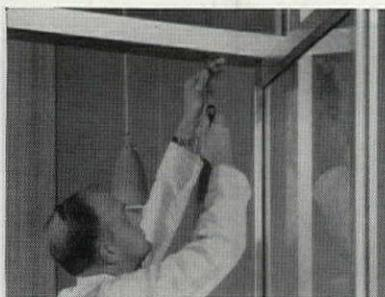
**EASIER SPEED ADJUSTMENTS** than with floor-check entrances. Kawneer Concealed Overhead Closer has two closing speeds, and has independent adjustments for both closing speed and latching speed. Also equipped with *spring tension adjustment* for severe wind conditions, independent of the hydraulic action of the other two speeds.
