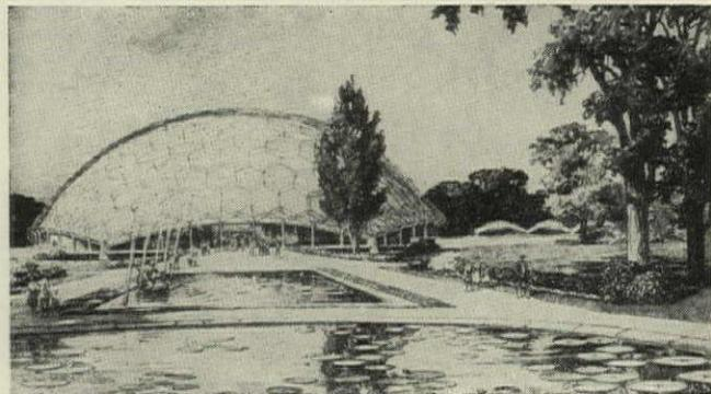
for giant greenhouse. Electronic-panel controls will be able to produce rain, mist, fog, arid air, or almost any other kind of atmosphere demanded by plants. Dome will be 175 ft in diameter at base and over 70 ft high at center, with no interior supports. Columbus Division of North American Aviation, Inc., will build structure.
