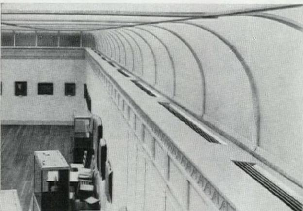
The photograph above illustrates an Anemostat Straightline Air Diffuser installation in the gallery design of the Sterling and Francine Clark Art Institute at Williamstown, Mass. The conditioned air is supplied through Straightline Diffusers located on all four sides of the gallery. The diffusers not only draftlessly introduce conditioned air into the gallery, but also blend into the architectural design.
