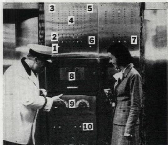
dually operated elevators has come the need for visual panels that portray the automatic operation of all parts of the system. These are under the supervision of a lobby attendant who may control the automatic program-selector and make occasional adjustments in the service (*Figure 6*). The conversion of many manually operated elevator systems to centralized automatic operation has produced economic comparisons that are highly
