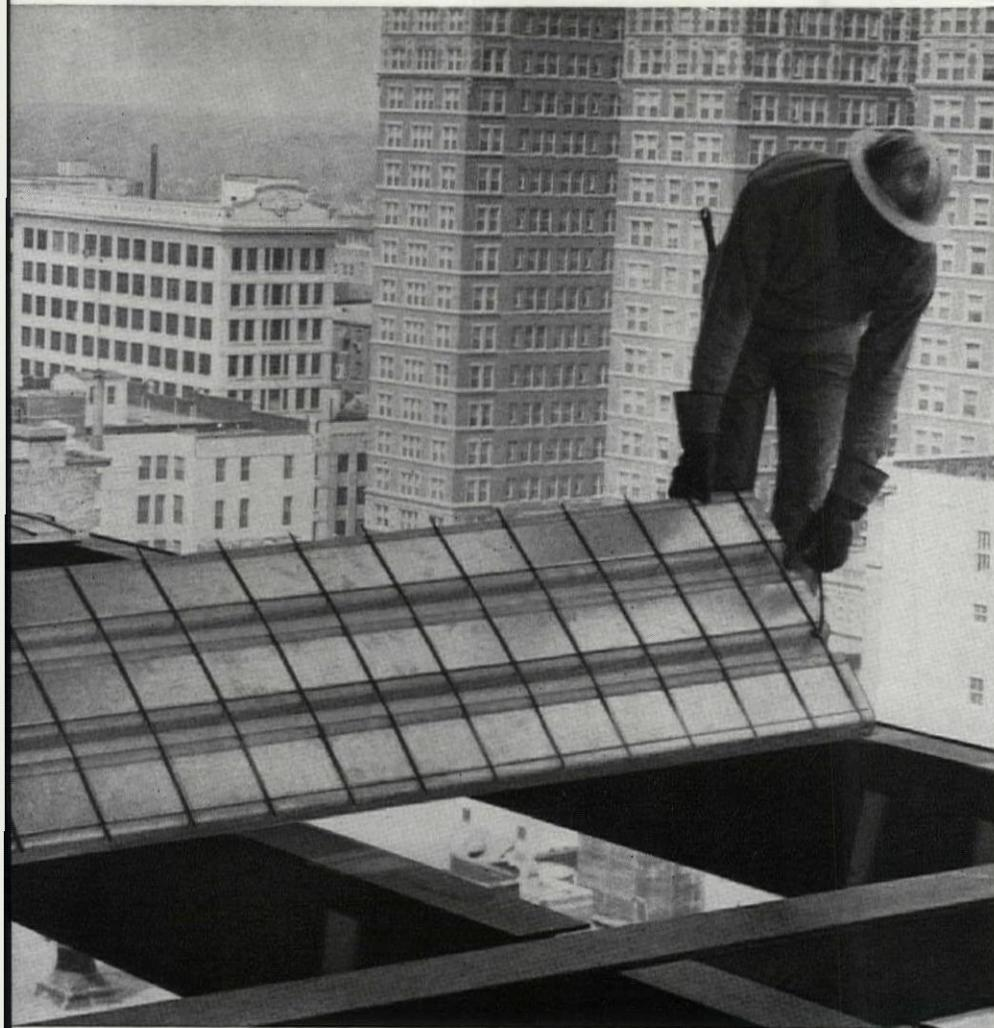
**PLACING E/R COFAR IS FAST, EASY.** Choice of 1-, 2-, or 3-cell units. Long spans (up to 14'4") mean less framing, lower costs. E/R Cofar units permit future wiring without necessitating a network of cells under the entire floor.
