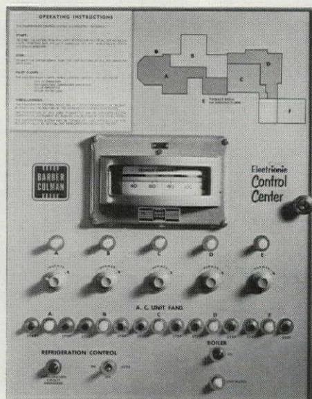
Figure 7—Electronic control center for large residence (below). Temperature control point for any zone thermostat can be reset by changing position of appropriate control dial below.
