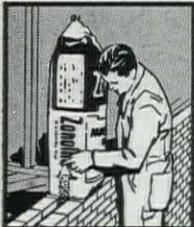
New Zonolite Water-Repellent Masonry Fill Insulation pours freely from light-weight bags, fills 100% around wall ties, conduit, etc., won't settle, sag or ball up; retains initial efficiency for the life of the wall itself.
