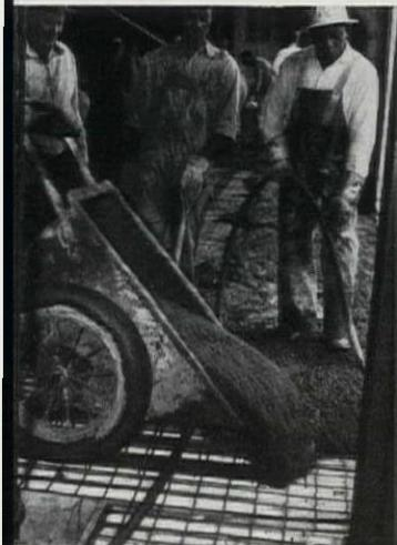
**GRANCO PRODUCTS PROVIDE FORM BASE** for concrete. Unobstructed work area speeds concreting. No wood forms. No wasted fill. Reinforced concrete construction. Granco ducts are available in a number of widths and gages to help you meet various load conditions.
