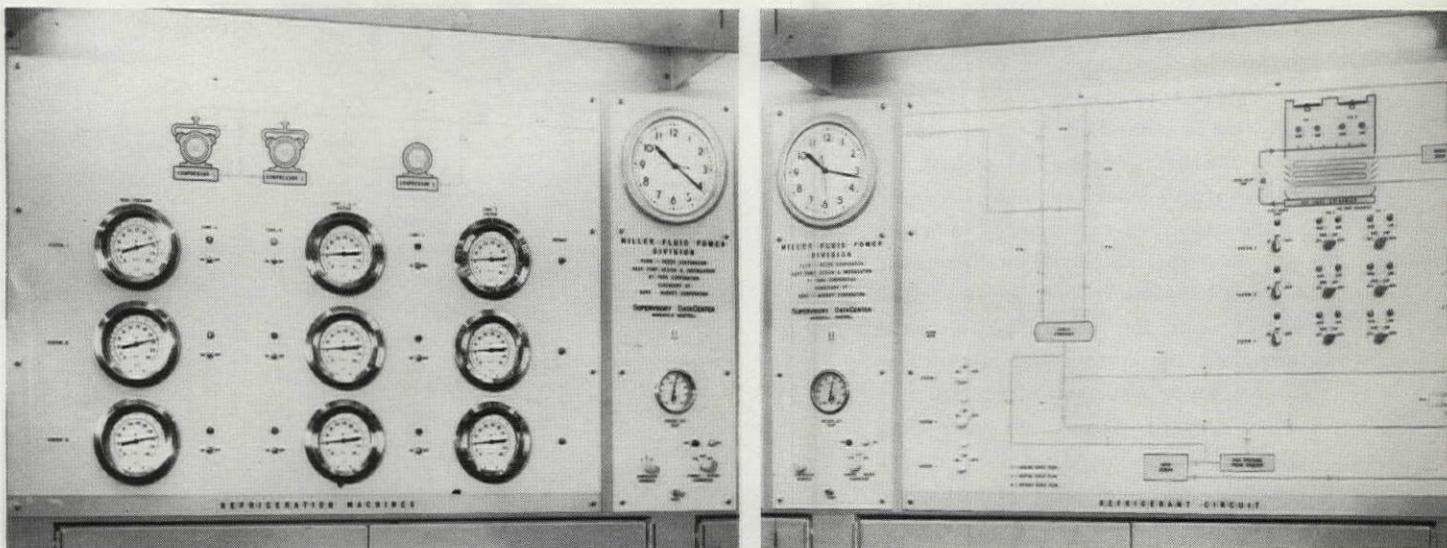
Figure 3—Control panels for Miller Fluid Power Division, Flick Reedy Corporation, Bensenville, Ill. Refrigerant circuits are identified on right panel; head and suction pressures for the three systems of refrigeration are indicated on dials at left.
