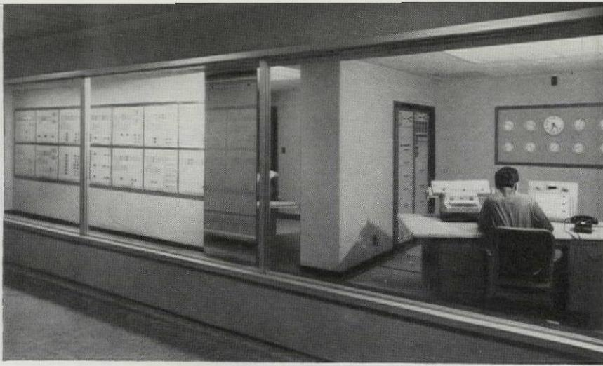
Figure 2—Linked to highly sensitive thermostats located throughout the building, this control center at the Queen Elizabeth Hotel, Montreal, enables one man—shown at control desk—to supervise and regulate the building's entire indoor climate.
