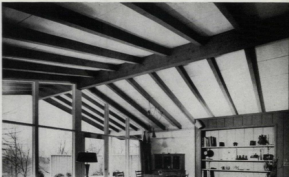
*Insulating roof-deck slab is nailed directly to beams (right). Built-up roof or asphalt-strip shingles can be applied over roof-deck slab. If latter is used, 2" or 3" thick roof-deck slab is recommended. After felt and tar are applied to slab, shingle application begins with installation of starter strip. Then, first course of asphalt-strip shingles is nailed down (below). Open-beam ceiling (top) has exposed under sides of insulating roof-deck slabs.*
