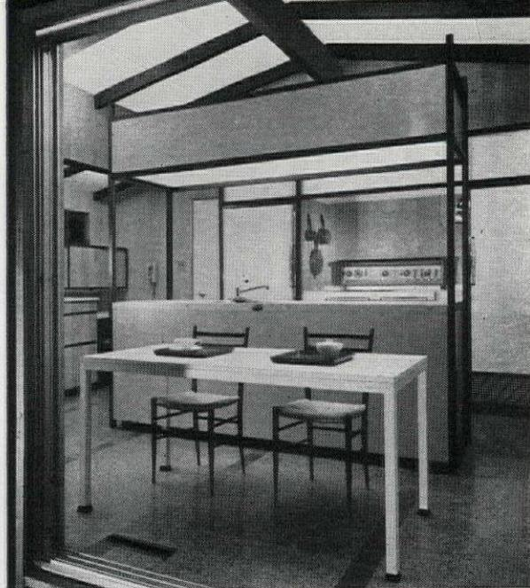
Home is designed on 3' module with four roof heights. Highest is over the living room.
