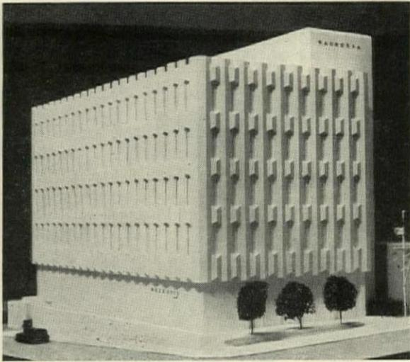
● Castellated Wachovia Bank and Trust Company Building in Wilmington, N.C., has exterior facing of precast-concrete panels, prism-shaped with textured surface of quartz. Light will reflect from angled spandrels differently at different times of day, causing quartz to sparkle. Designed by A.G. Odell, Jr., & Associates, with Ballard & McKim as Associate Architects.
