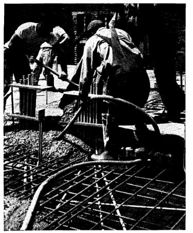
**ELECTRUNITE'S** tightly adhering galvanized coating protects against corrosion, won't peel, chip, or flake off during bending. Millions of feet have been successfully used in slab concrete installations over the past twenty-five years.
