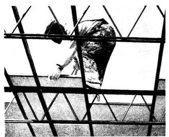
New PYROTONE Formboards for use with PYROFILL Gypsum Concrete Roof Decks are designed especially for exposed ceilings. As formboards are installed, an attractive ceiling is built–quickly and easily. PYROTONE Formboard and PYRO-FILL Gypsum Concrete are both manufactured by U.S.G.
