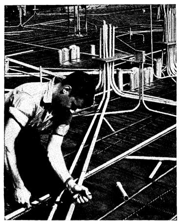
**GOOD INSTALLATION PRACTICES** call for tying Republic ELECTRUNITE E.M.T. to steel rebars. With steel conduit there is no danger of galvanic action.
