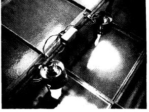
Figure 4—Customary installation design in paintings is with incandescent and "cool" white fluorescent lamps mounted over a center-of-room **T**-grid of tempered water-white glass (left). Detail of specially designed incandescent "scoop" fixtures (above).
