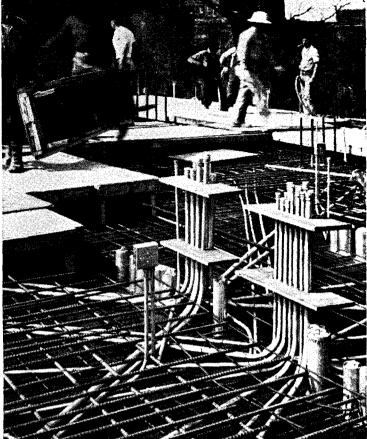
ELECTRUNITE"INCH-MARKS"<sup>®</sup> and "GUIDE-LINES"<sup>®</sup> help make compact stub groupings. The strength of steel provides protection against damage.
