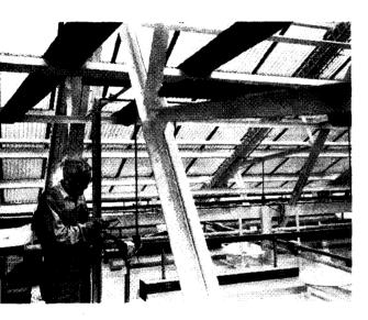
Figure 1--Presently being reconstructed, Wing E of the Metropolitan Art Museum will ultimately have an electrical and lighting installation comparable to Wing J. Workman (above) connects two conductors above the  $\mathbf{T}$ -grid in Wing E.
