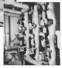
International Minerals and Chemical's new administration and research center, Skokie, Illinois, has been described as "engineered for thinking." In keeping with that objective, twenty-two *quiet* B&G Boosters were selected as the pumps for the heating circuits of the four buildings and the snow melting panels.
