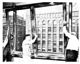
STAINLESS STEEL REVERSIBLE WINDOWS, here being installed at the Morton Salt Company Office Building, Chicago, Illinois, were fabricated by Republic's Truscon Division. Architects: Graham, Anderson, Probst & White, Inc. Contractor: Sherman Olson, Inc.
