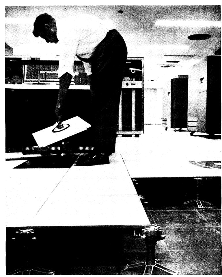
Complex network of cables seen during installation of a large-scale IBM computing system will be completely concealed by an elevated floor of Alcoa Aluminum. This installation is at the office of United Medical Services, Inc. (New York's Blue Shield).
