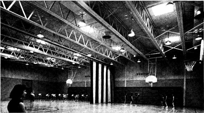
**GYMNASIUM** incorporates both Tectum roof deck and sidewall panels for maximum insulating and acoustical value. Roof deck is  $2\frac{1}{2}$ " thick; sidewall panels are 2" thick with neat beyeled edges and tongue and groove joints. Four walls and a ceiling for effective sound control in an area where noise can be a problem during study periods.
