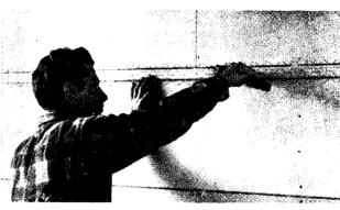
KEYSTRIP can be used as a reinforcement for plaster in a space too narrow for strips of gypsum lath. A full bond of Keystrip to the plaster is assured. Keystrip also adds strength to points of stress above doors and windows.
