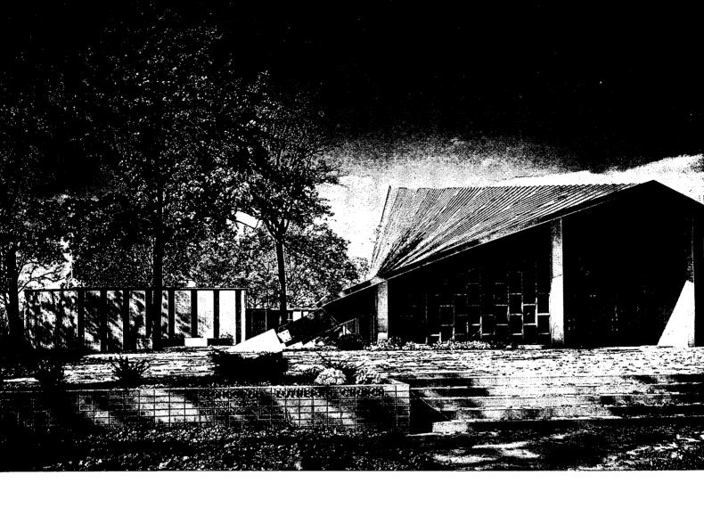
The roof, a dominant element because of its size and shape, demanded careful surface treatment. Sheet copper with batten seams arranged in an interesting triangular pattern added architectural interest. When oxidized, its blue-green will be the principle color of the exterior,
