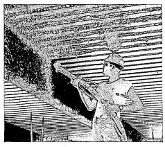
Fire-Shield Plaster is sprayed directly to the steel deck. It adheres instantly, and when dry it forms a bond that will withstand a direct 400 pound pull.
