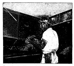
Beam Furring Clips attach metal lath to steel beams with a gentle tap of the hammer. They eliminate costly bracketing, and cut labor costs in half.
