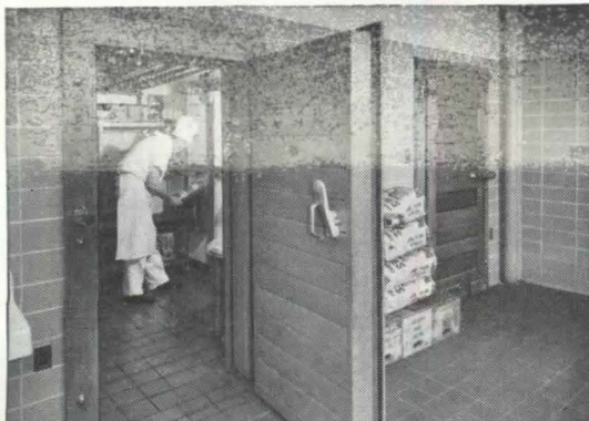
Both walk-in refrigerators are insulated with Styrofoam.
