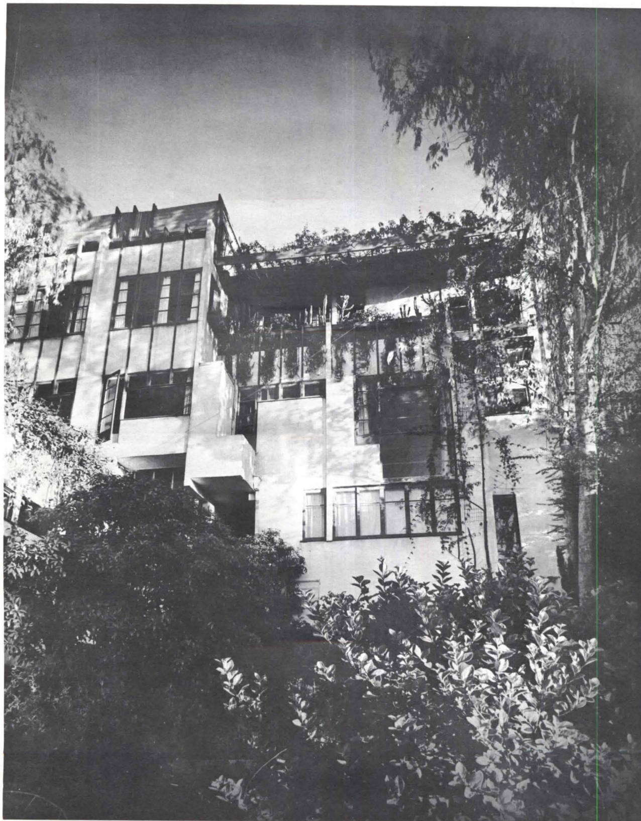
In the Sachs apartment house, Los Angeles, 1928, Schindler turned from concrete to studs and plaster—his first attempt to develop his own vocabulary within standard framing. Each apartment had an entrance from the street and a glass wall facing a living porch.
