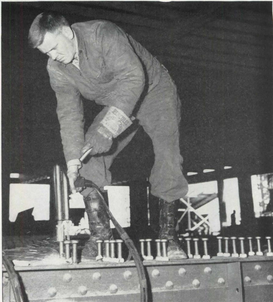
In welding stud to top flange of steel beam, ceramic ferrules containing annular openings—which control the vapor products of welding—are used. These are subsequently knocked away.
