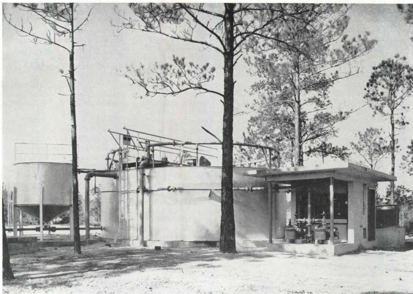
1 Rectangular-type aerobic digester (above)—serving 300 people—is suitable for small centers not accessible to municipal sewer lines. 2 This 30' diameter steel tank (below)—applicable to remote installations—handles flow of 40,000 GPD, has 24-hour aeration period.
