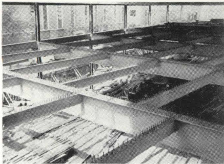
Typical steel floor framing system with welded studs placed on both beams and girders.
