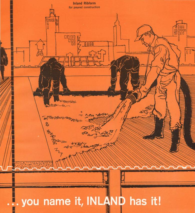
In concrete-over-steel construction, Inland Ribform supports wet concrete with minimum deflection. Rigid sheets are quickly and inexpensively attached to supports — in place, they provide a safe work platform for crews.
