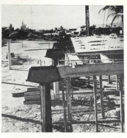
signed with a cast-in-place deck slab. Prestressedconcrete piles driven through the fill material were designed for point bearing on the coral ledge. The piles were designed to stand cs columns, the upper end of the column being cast-in-place in an adjustable steel form. Reinforcing steel for the upper section of the
