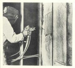
odorless. Spraying is done with a high-speed gun that mixes the chemicals, atomizes them, and forces them out of the gun. The insulation has a K factor of 0.15 at 75 F. and a 2" layer is equal to or better than 3" of the best conventional insulations. Additional advantages: a permanent monolithic seal devoid of seams; excellent soundproofing characteristics; and high moisture-vapor impermeability almost equal to plastic film. Dayton Industrial Products Company Division, Dayco Corporation.
