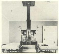
mounted emergency station makes it possible to bring all supply lines oxygen, vacuum, and electricity—directly to bedside without crossing floor. Beds can be located in center of room for improved circulation. Unit provides complete facilities for two patients. National Cylinder Gas Division, Chemetron Corporation.
