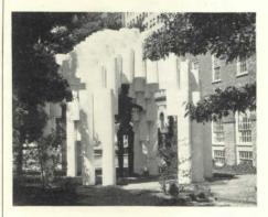
a wooden frame extending four feet into the ground for protection against high winds. For weather-proofing, the tubes were treated with a mixture of waterglas and paint. For news of RISD's Rockwell K. DuMoulin, see page 58.
