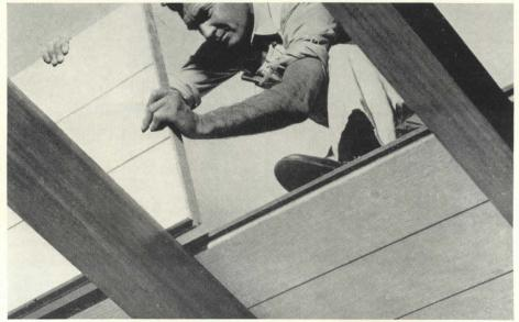
Insulating roof deck may be used in exposed beam construction.
