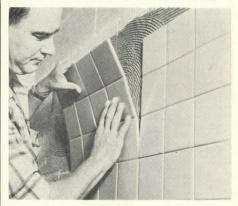
special cement. Sheets do not buckle in handling, yet mesh can be easily trowel-cut. Mortar, mastic, or mortar mix are suitable for installation, coming in contact with 70 percent of the tile surface. Soaking is not necessary. Stylon Corporation.
