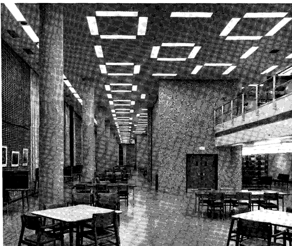
Day-Brite Troffers with Cleartex® Plastic Lens Panels deliver 73 footcandles of illumination to reading areas.
