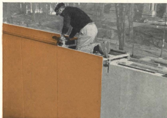
INSTALLING THE BRONZE "SKIN" over one of the cross members which run across the roof.
