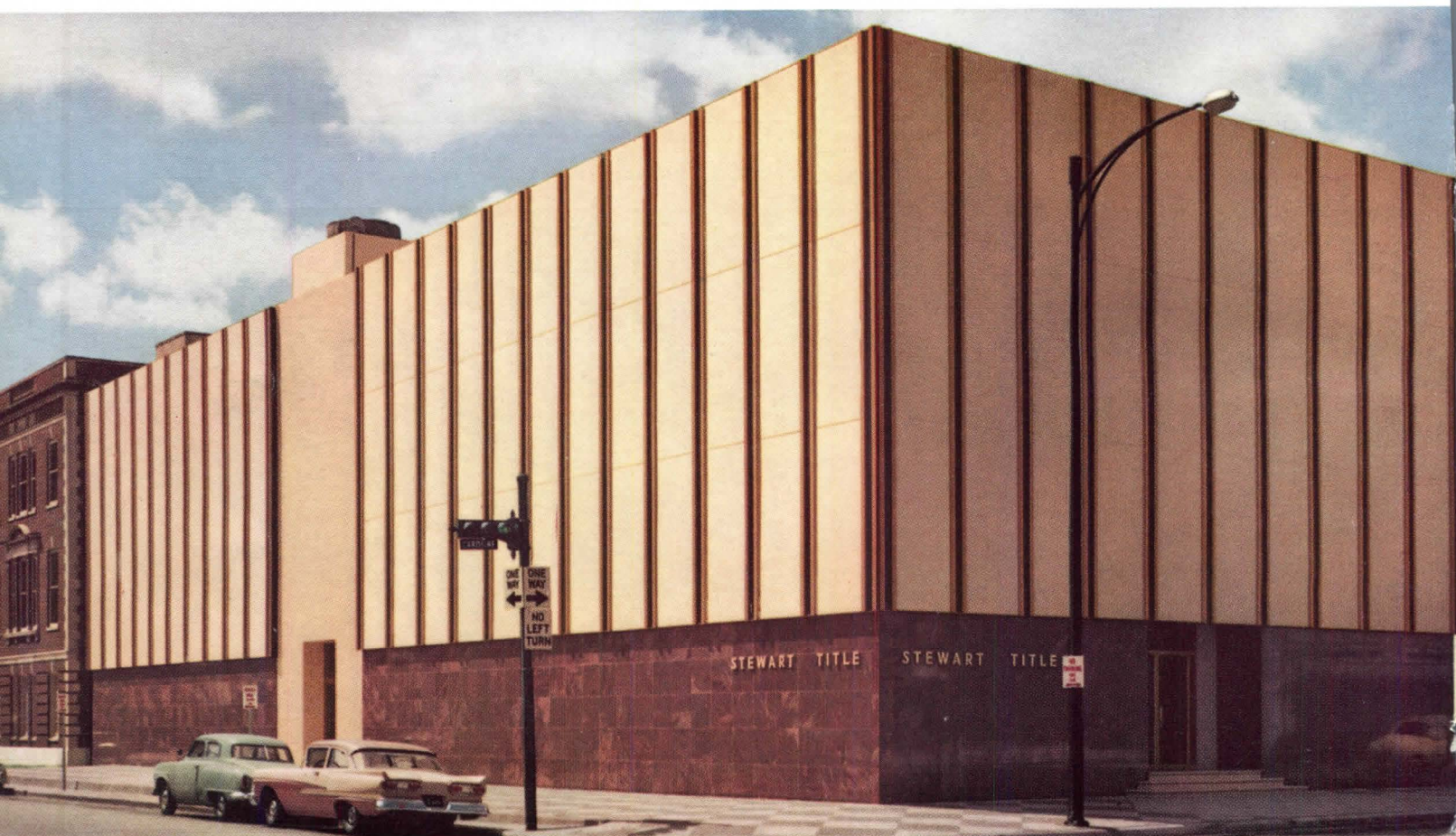
Floating curtain wall facade of the remodeled Stewart Title Guaranty Company Building is composed of three 4' x 10' cream Glasweld panels in each channel. Renovation was designed and installed by Architectural Metal Erectors and Brososke Engineering and Manufacturing Corporation. Consulting Architect: John Freeman, Jr.
