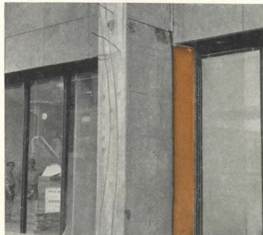
UPRIGHT CONCRETE GIRDER before covering with bronze "skin." The Revere Muntz Metal used was in thicknesses of \frac{1}{4} " and \frac{3}{16} ", ranging up to 40" in width by 11' 11" in length.
