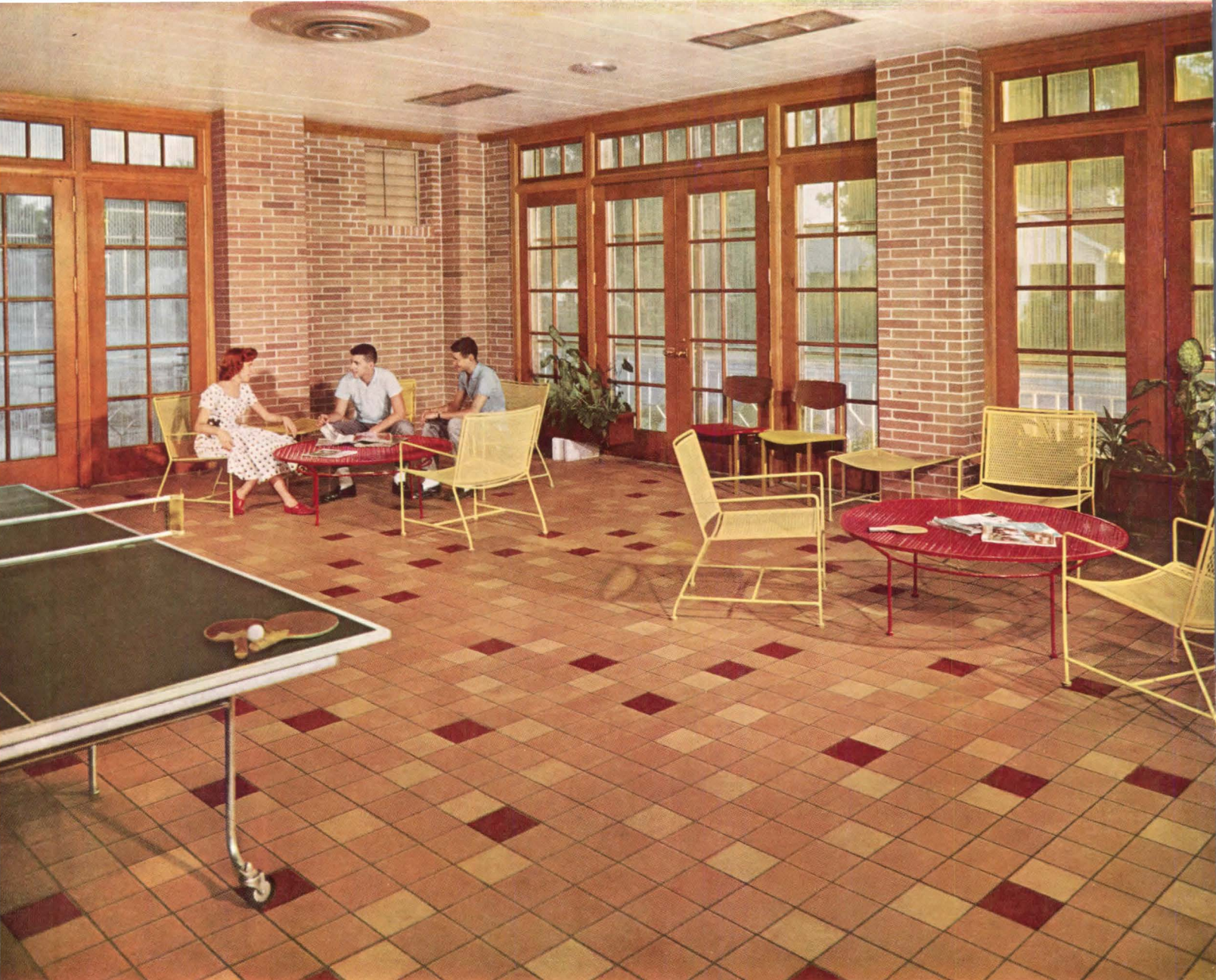
Tuscaloosa, Ala., Y.M.C.A. Recreation Room. Floor is 6" x 6" x 1/2" Murray Quarry Tile in Canyon Red, Golden Glow and Sahara. Architect: Wilmont C. Douglas & Carl M. Moseley. Tile Contractor: Sealy & Jehle Tile Co. Plate 422.
